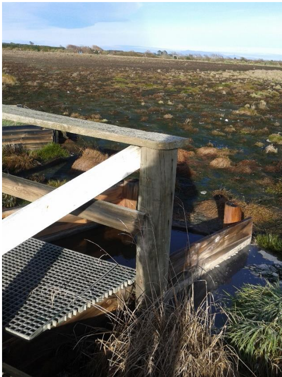
Figure 2: Waste water anaerobic pond (first part of the waste water treatment)
