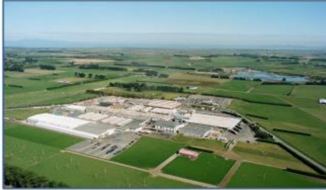
Alliance Lorneville meat processing and export plant with wastewater treatment ponds in the background.
