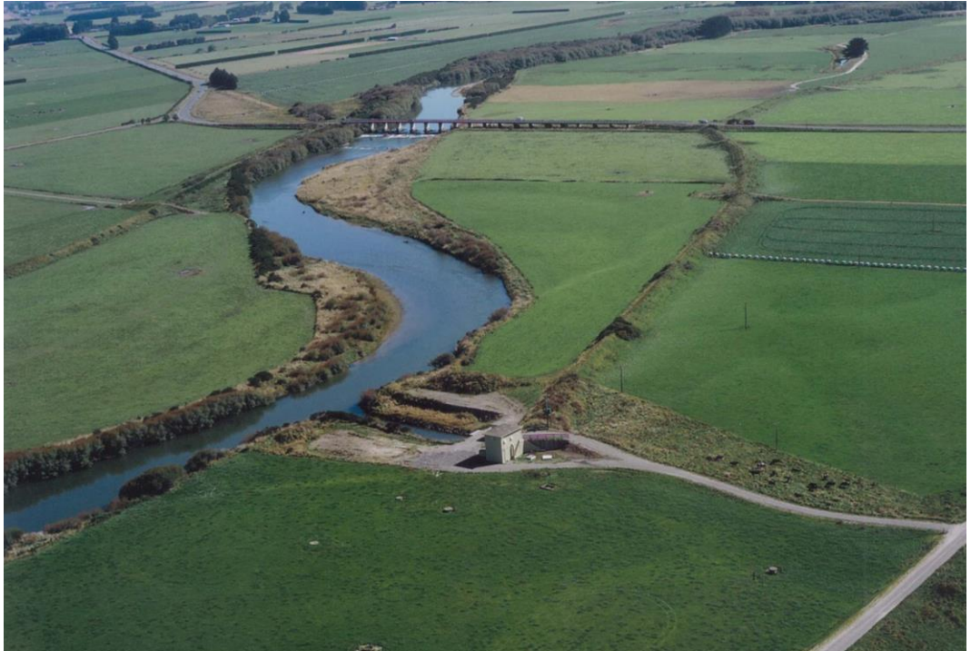
Figure 10: View of the Alliance water take and Wallacetown Highway Bridge.
