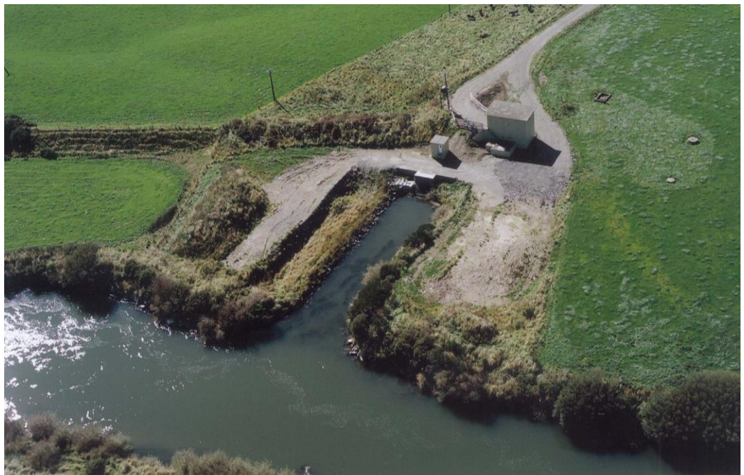
Figure 9: View of the Alliance water take from the Oreti River.
