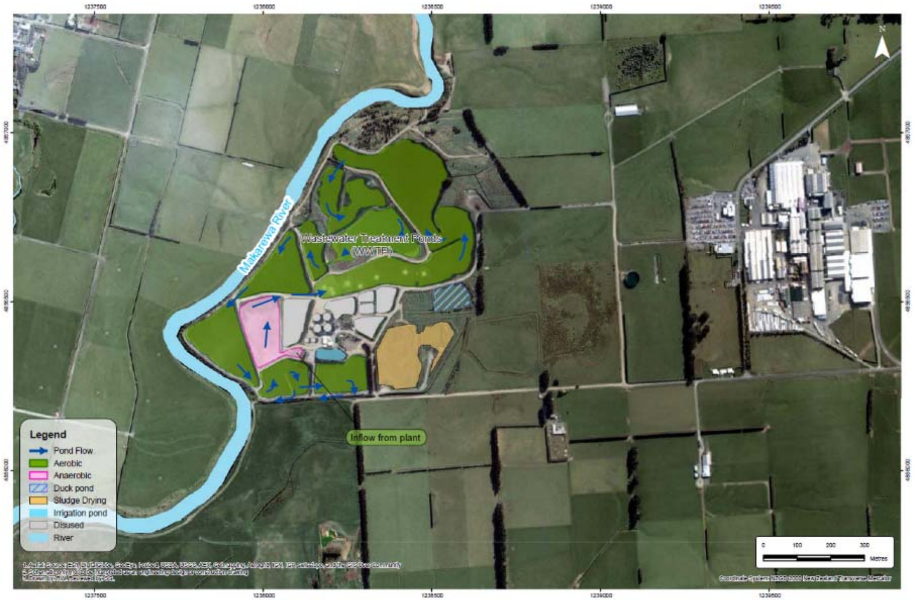
Figure 2 in Attachment R to the AEE (as referenced in the evidence): Wastewater Treatment Plant.
