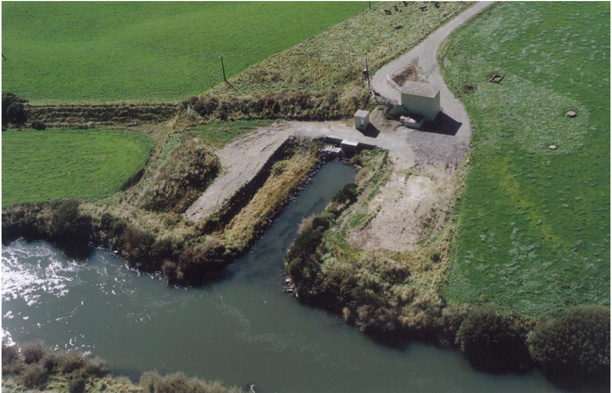
Figure 3: View of the Alliance water take from the Oreti River.
