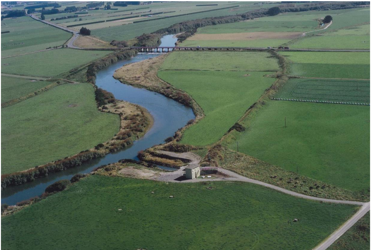
Figure 4: View of the Alliance water take and Wallacetown Highway Bridge.
