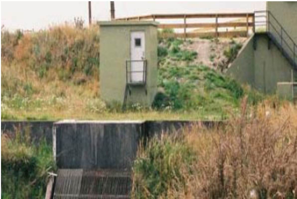
Figure 25: View of intake structure.
