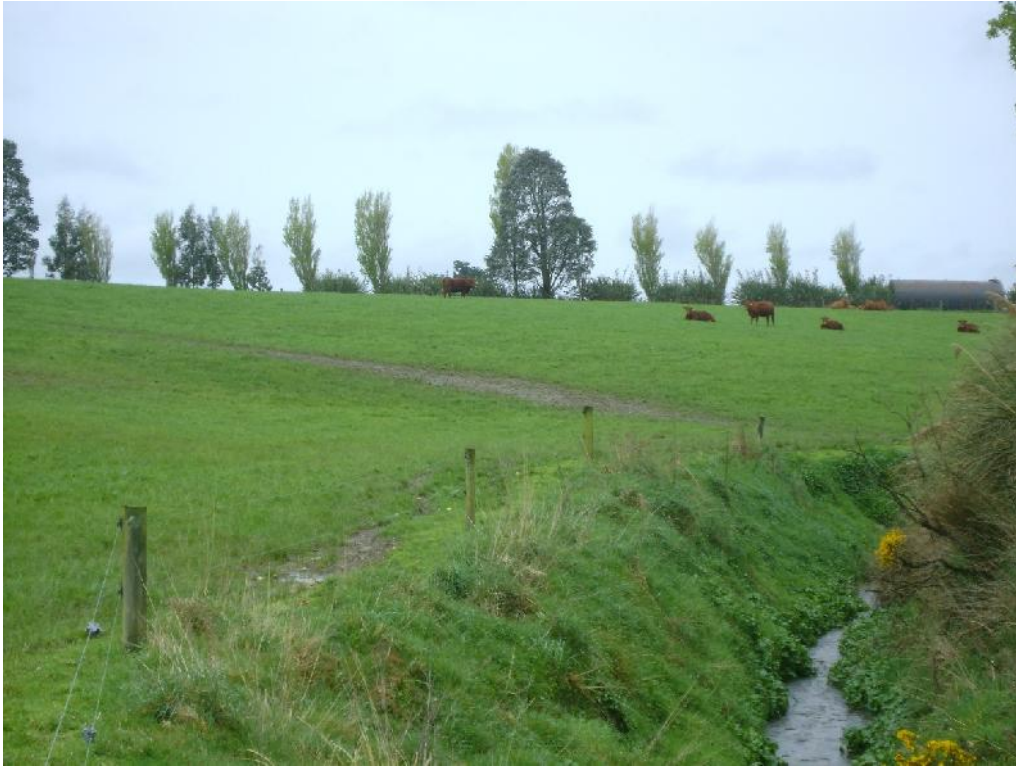
Figure 5: McMillan Creek - unplanted edge to facilitate ES stream clearing works looking south from bridge
