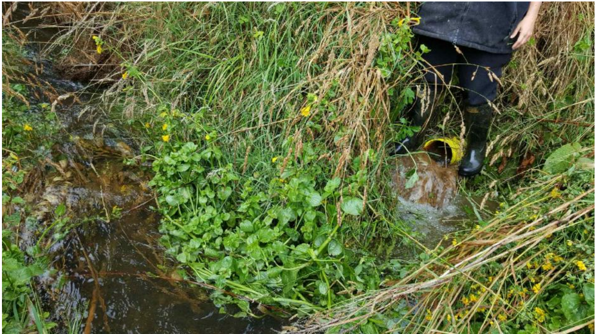
Figure 2: Tile Drain Outlet to McMillan Creek
