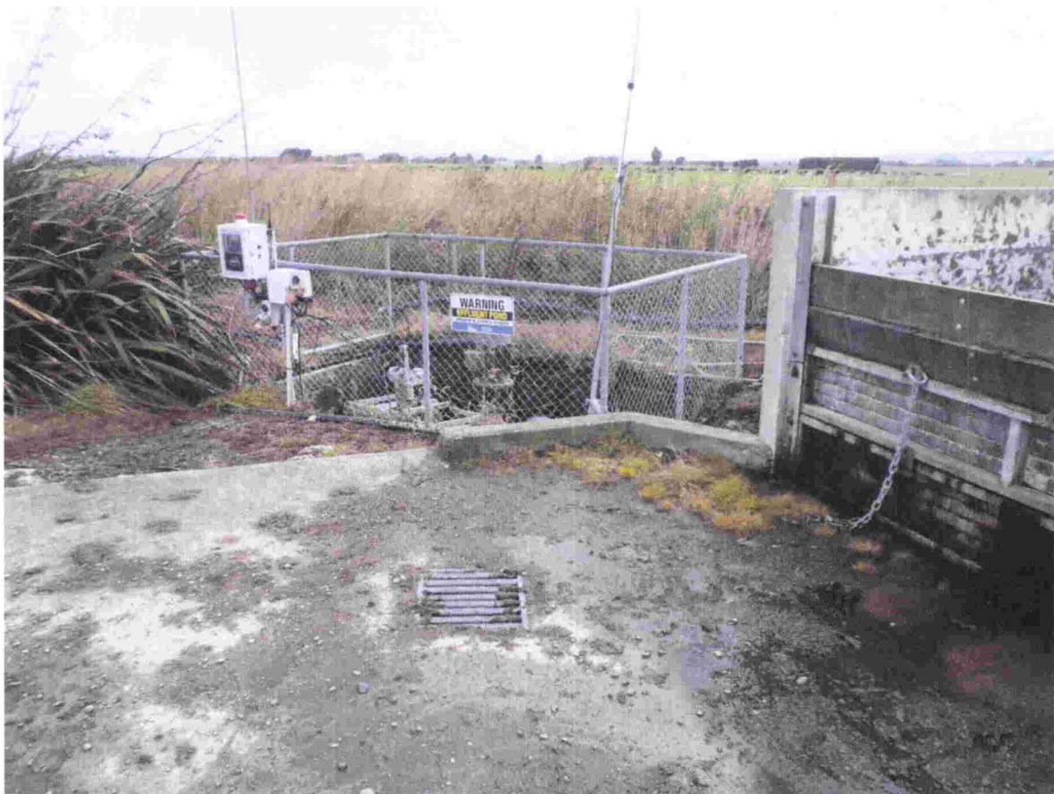
Pump sump and storage pond behind
