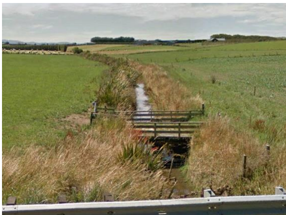
Figure 1 Drain looking north east from Winton Lorneville Highway (Google Earth, 2017)
