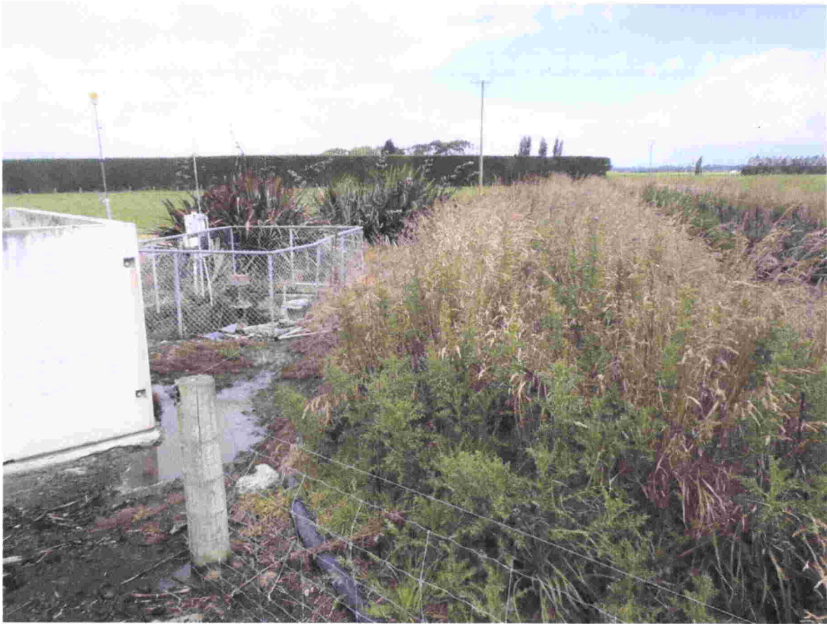
Pump sump and storage pond
