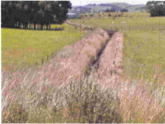
Figure 2 Drain facing north east from Winton Lorneville Highway (Google Earth, 2017)
