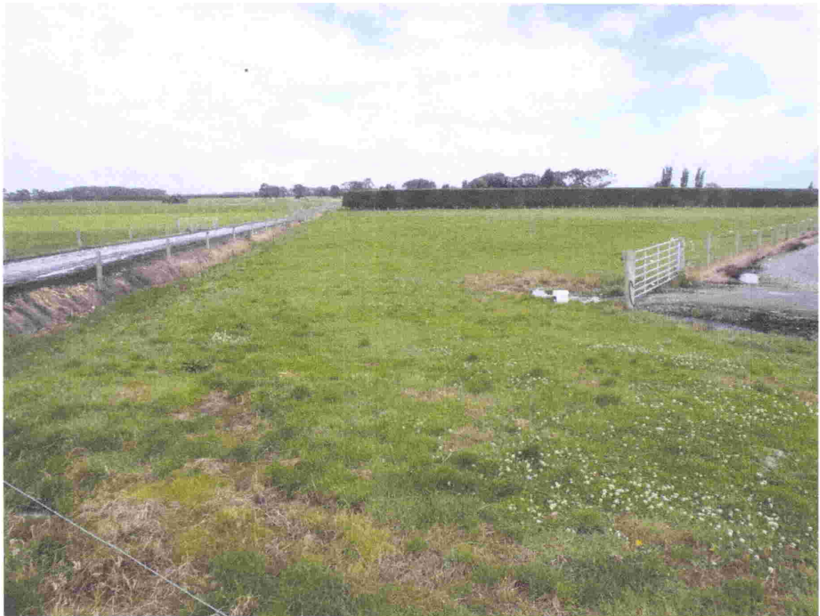
Looking west along line of new feed pad
