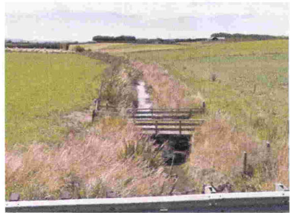
Figure 3 Drain looking north west from Winton Lorneville Highway (Google Earth, 2017)
