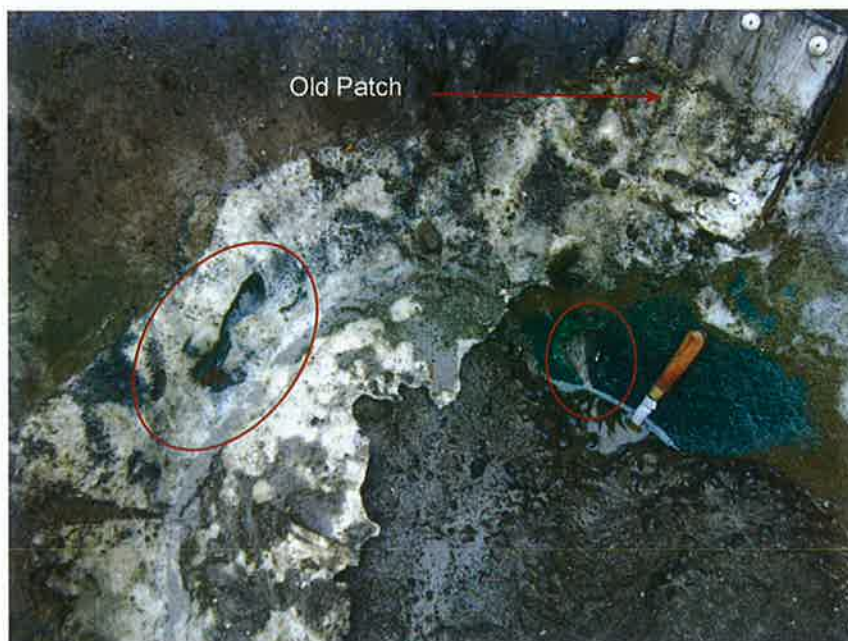
Figure 6. damaged sump.
