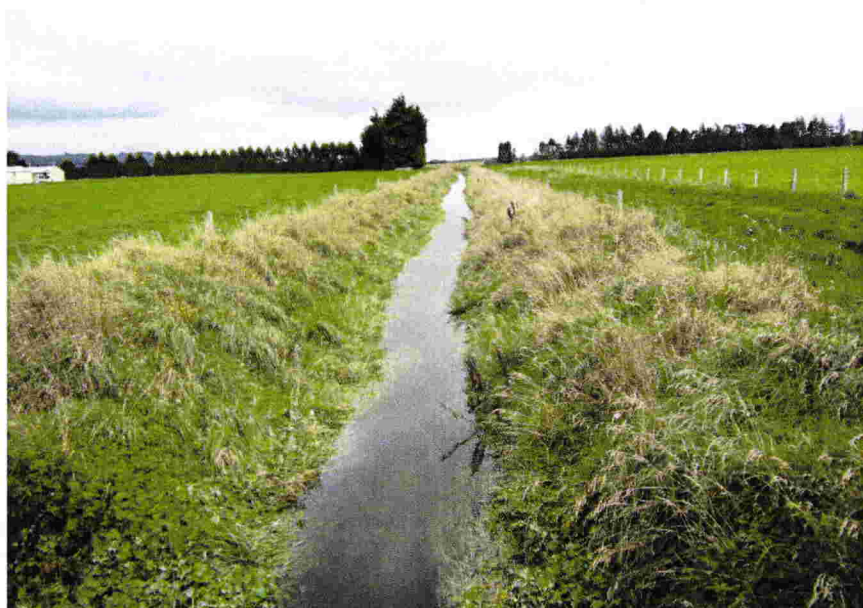
Main south drain
