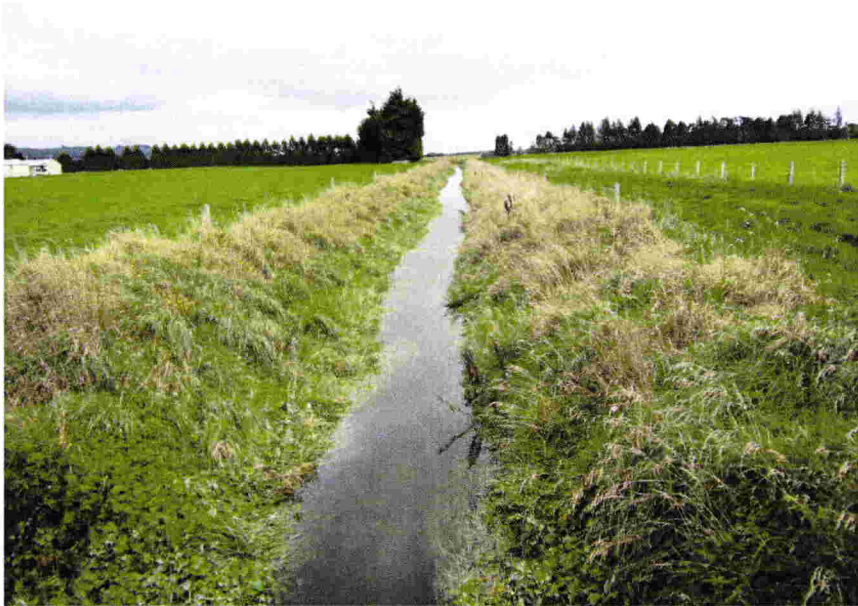
Main south drain
