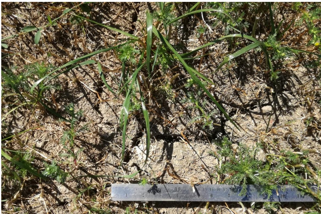
Figure 1. Cracked soil at Site 1.
