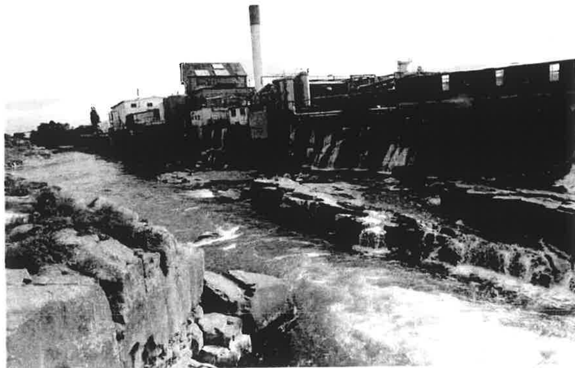
Figure 7. Alliance Matura downstream of the falls showing flows across the rock shelves as a result of the hydro race discharges
