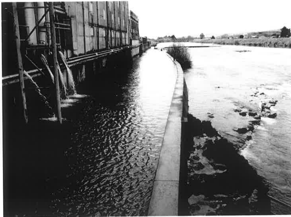
Figure 3: Existing Hydro Race
