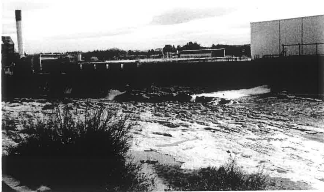
Figure 6. Alliance Matura showing flows from the headrace through sluice gates and overflows
