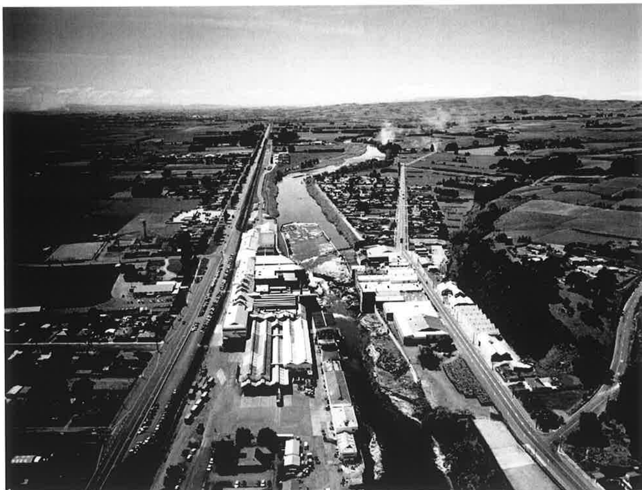
Fig. 2.1: The present day Alliance meat processing plant (left side of picture) and the Mātaura River with the Mātaura Falls and the upstream U-shaped diversion weir.
