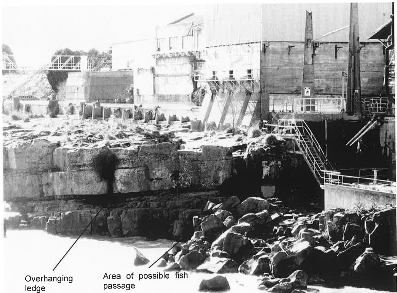
Fig. 4.1: The edge of Mataura Falls showing the eroded ledge and overhanging rock across the possible fish climbing routes. Note the one wetted area on the extreme right of the picture that provides a potential climbing route.
