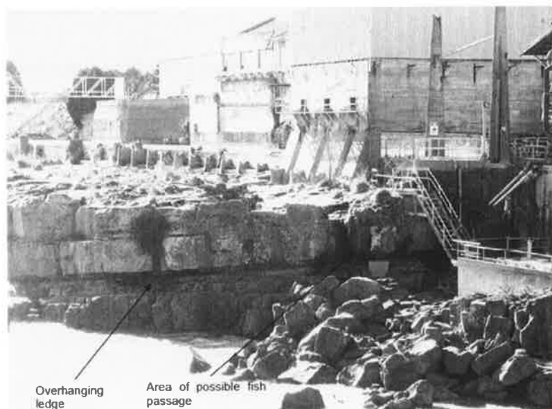
Figure 2-1: The edge of the Mataura Falls on left bank showing eroded ledge and possible passage route for elvers. From Allibone2007.
