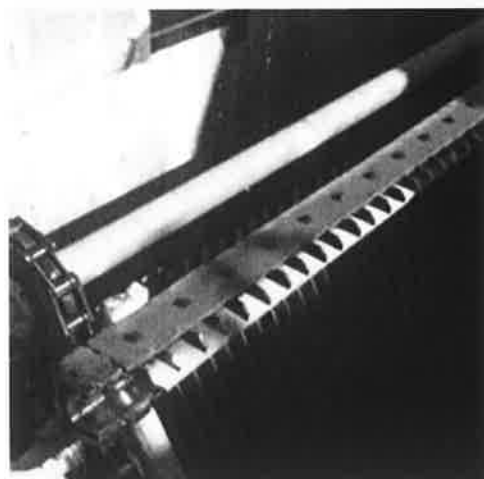
Figure 3-6: Trash cleaner bar progress up the screen. (Top) Rake bar reaching the apex of screen; (Middle) Rake at apex of its run; (Bottom) Rake on its way back down the screen. Note: If required in future it may be possible to make the rake bar more eel friendly by widening the rake blade and providing a backing plate and sides so as to produce a bucket that could safely hold the impinged eels
