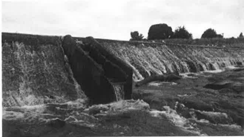
Figure 3-3: The Matura Weir summer 2017. Note salmonid ladder at centre weir. Photo courtesy Alliance.
