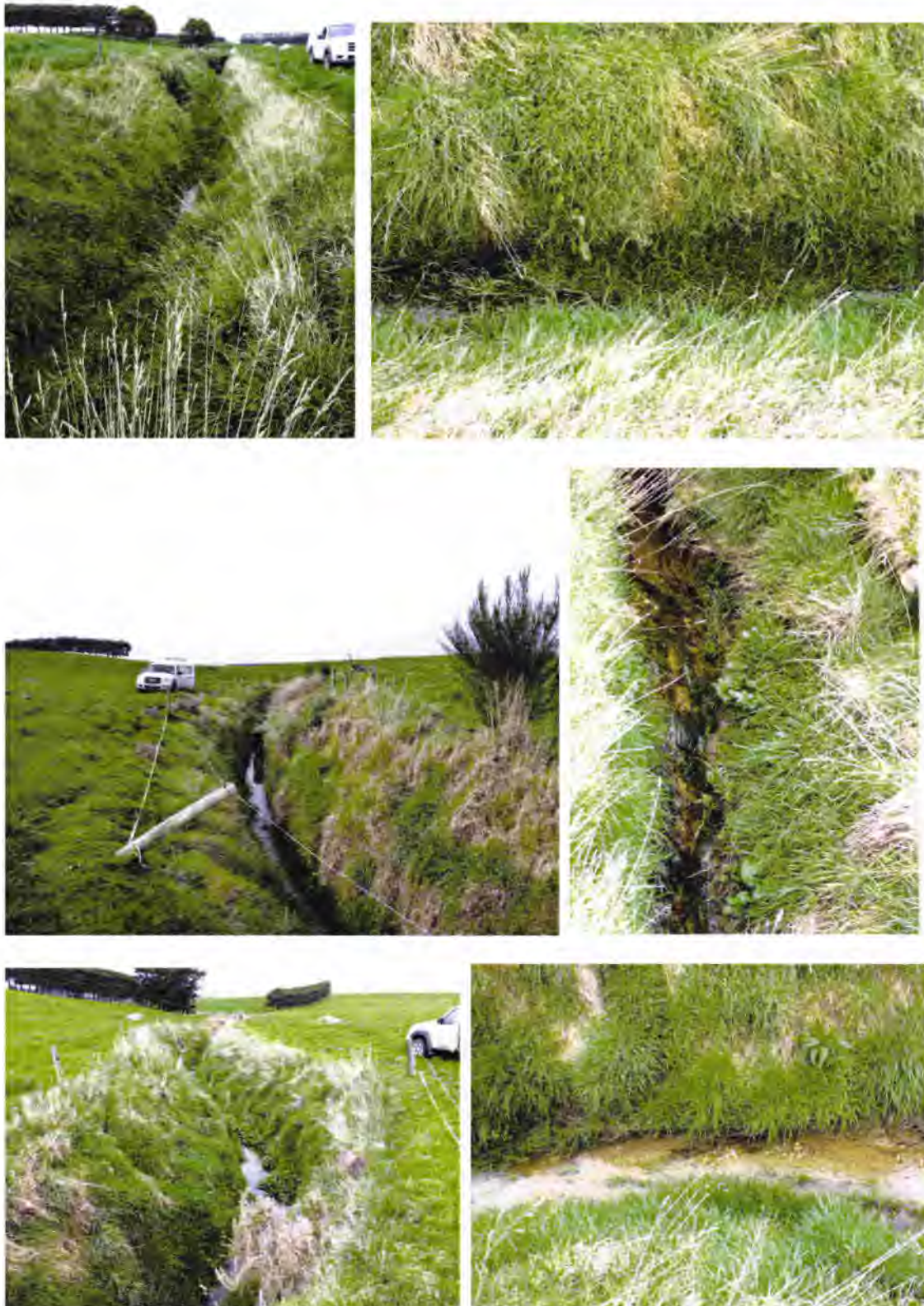
Figure 3 Top to bottom (upstream to downstream): Higham tributary sites – H1, H2 and H3.
