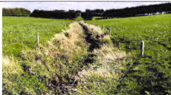
Photo 24 – Waituna Creek Eastern Tributary – Section Proposed to be Piped.
