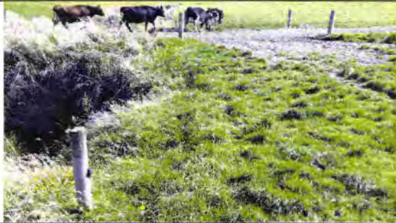
Photo 4 – Waituna Creek Planting Zone 2 – Slumped Area
