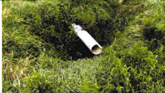
Photo 29 – Tile drain from Phiskie’s property entering small tributary
