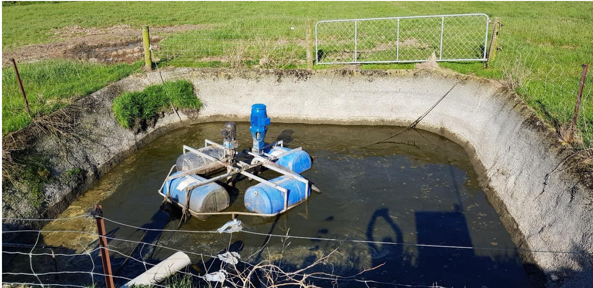
Figure 2: Concrete one-day pond
