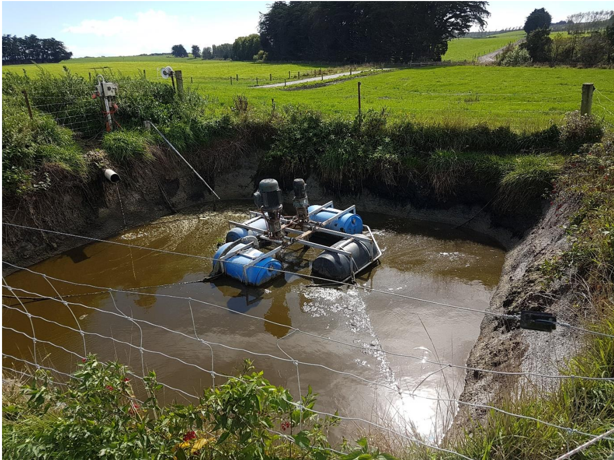
Figure 1: Photo of concrete saucer
