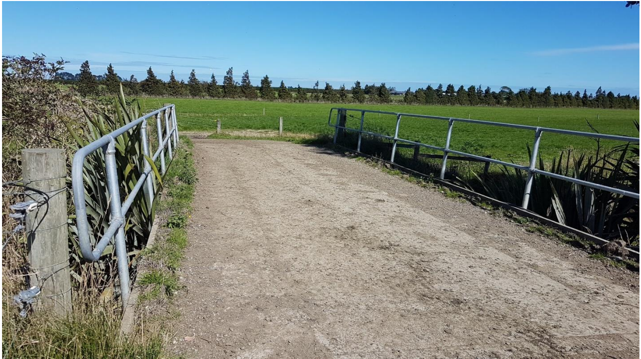
Figure 21: Photo of existing crossing on current dairy platform with barge boards to capture runoff
