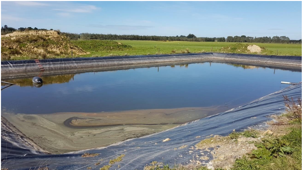
Figure 5: Effluent storage pond with HDPE liner
