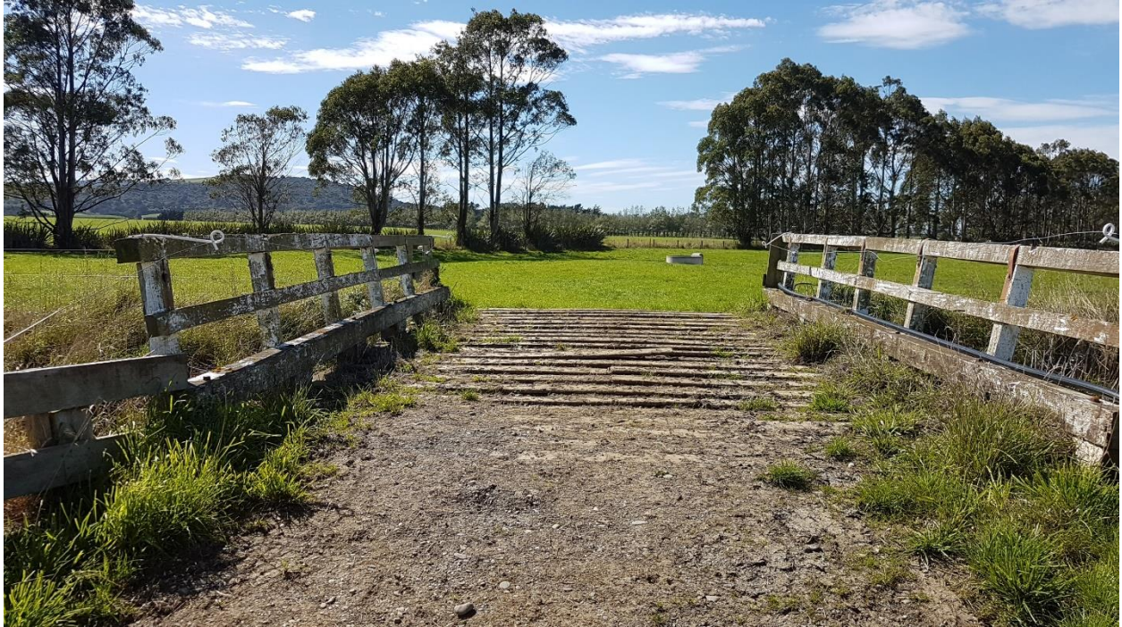
Figure 23: Photo of bridge crossing showing bargeboards and gradient to direct runoff to pasture
