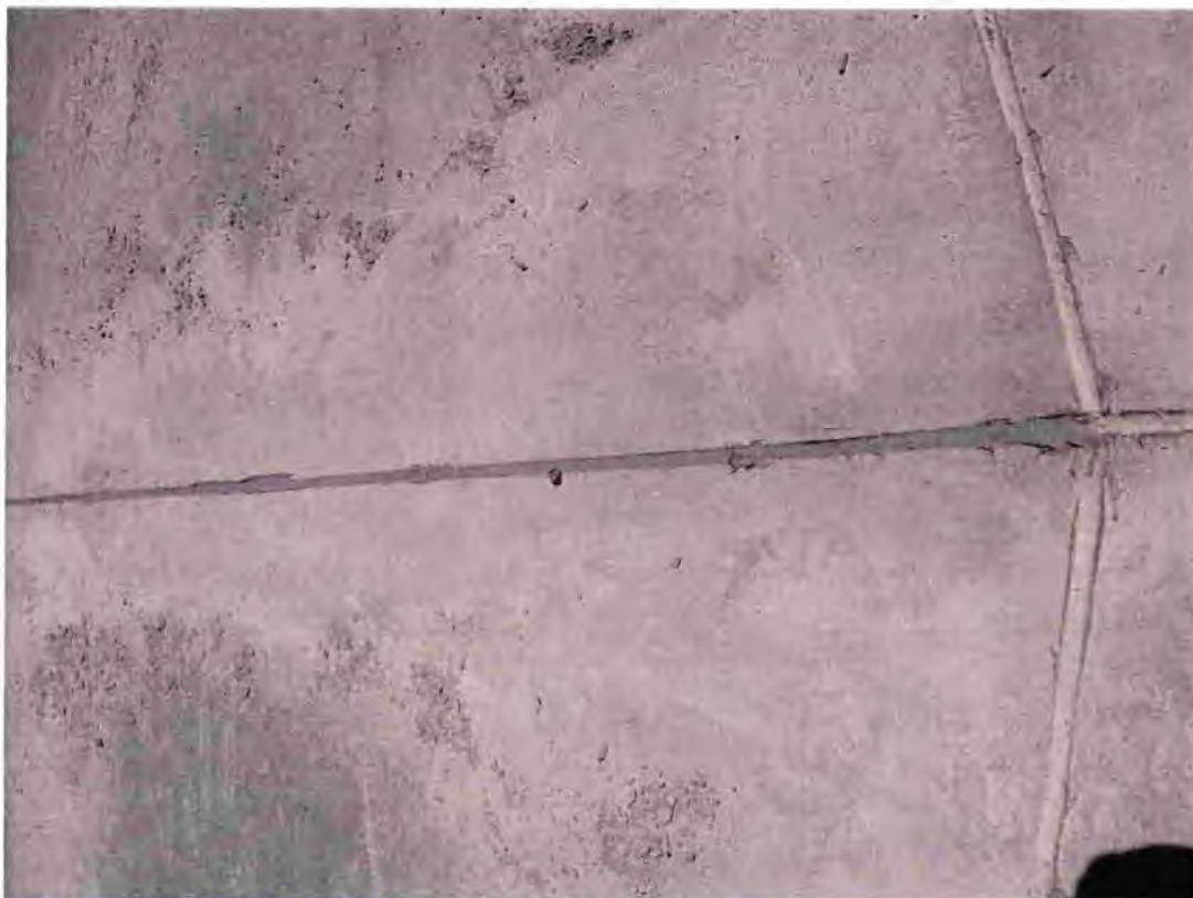
Final inspection – Control joints 15/02/2012
