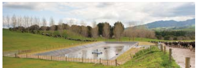
Ponds and storage facilities
