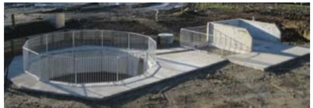
Sand traps and sumps
