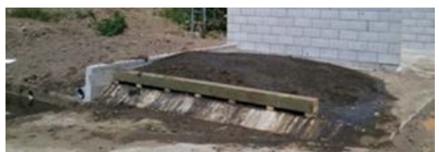
De-watering pads and solids storage bunkers
