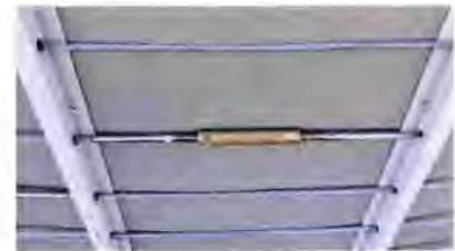
Swages and Turnbuckles used to connect wire rope
