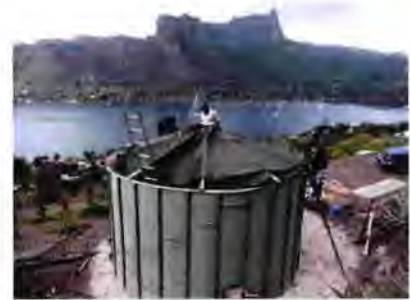
Roof Cover - PVC Aqualon Ripstock GRK 1000 UV inhibited, vermin and insect proof.
