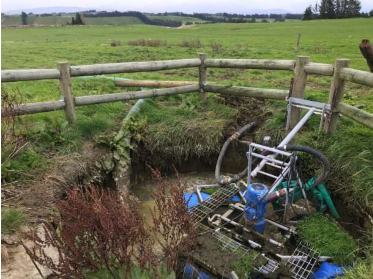
Figure 2: The pump sump near the dairy shed. This has been included in the revised Massey Pond Calculator as effluent storage.
