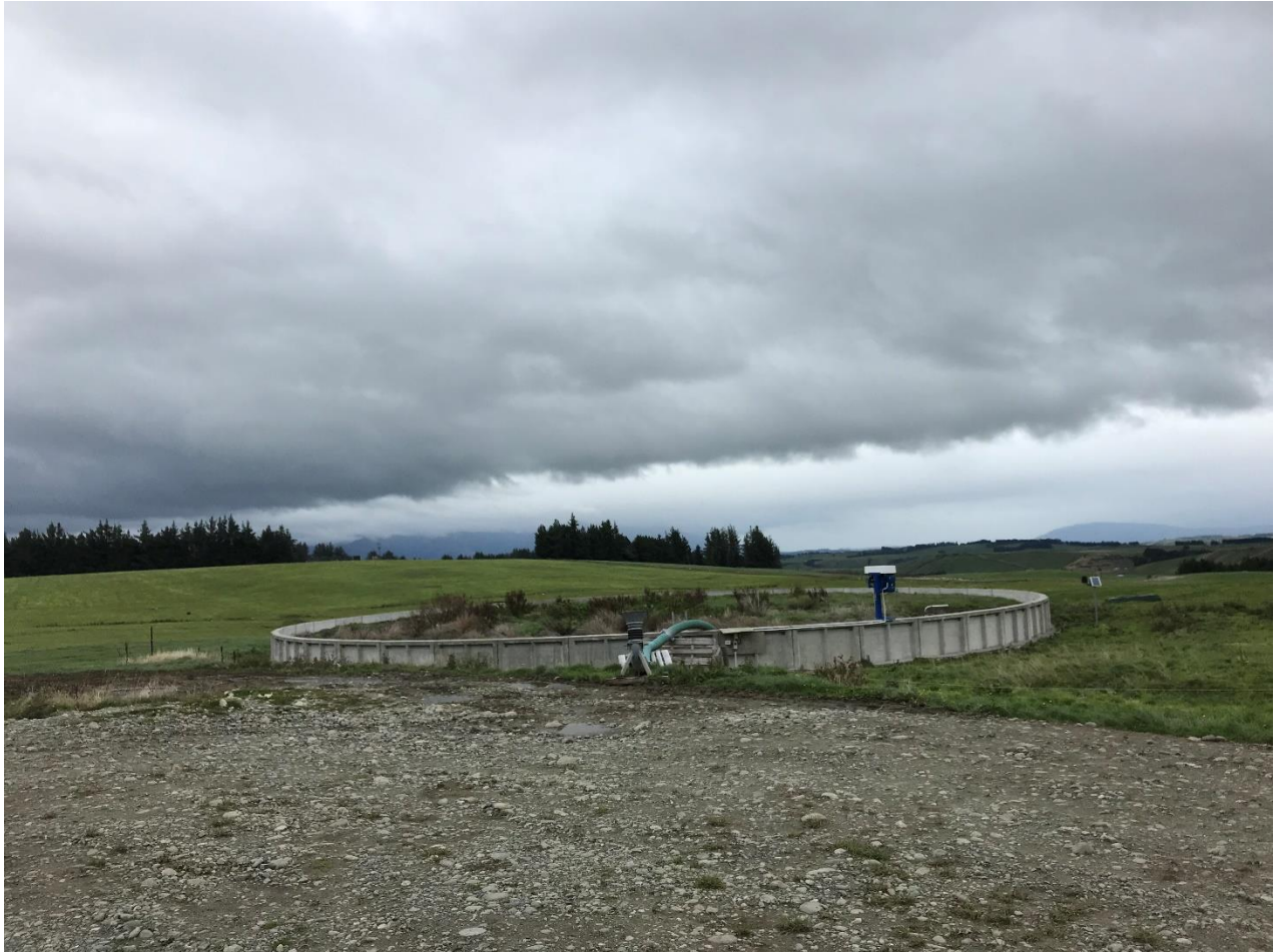
Figure 1: Photo of effluent storage tank looking out over property. The dairy shed is located down past the trees.
