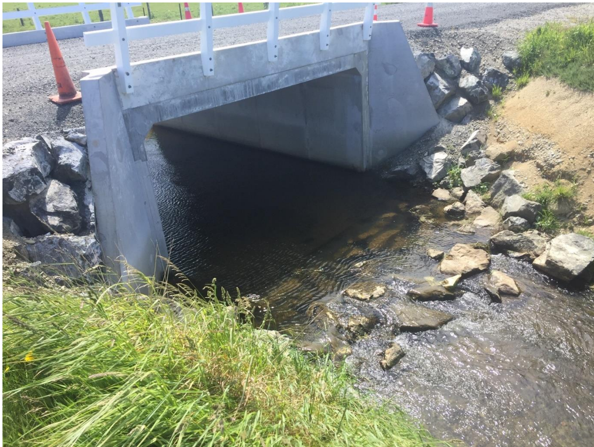
Figure 2: Waianiwa Oporo Road culvert downstream end.
