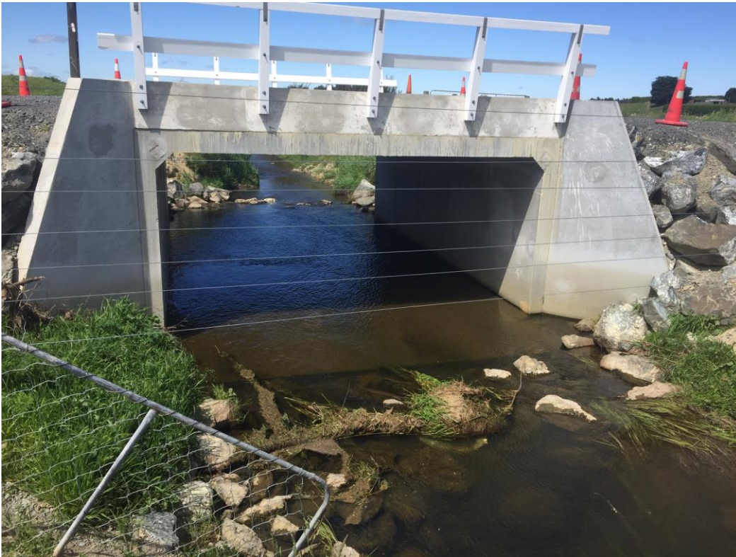
Photo 3: Showing rocks placed at each end of culvert.
