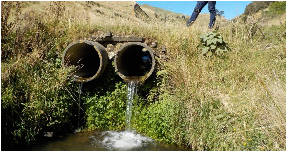
Figure 5: An example of a culvert fish passage barrier to all fish species.
