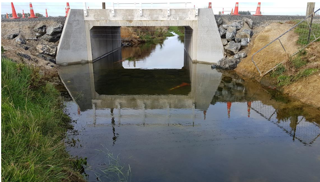
Photo 1: Looking downstream through culvert following installation
