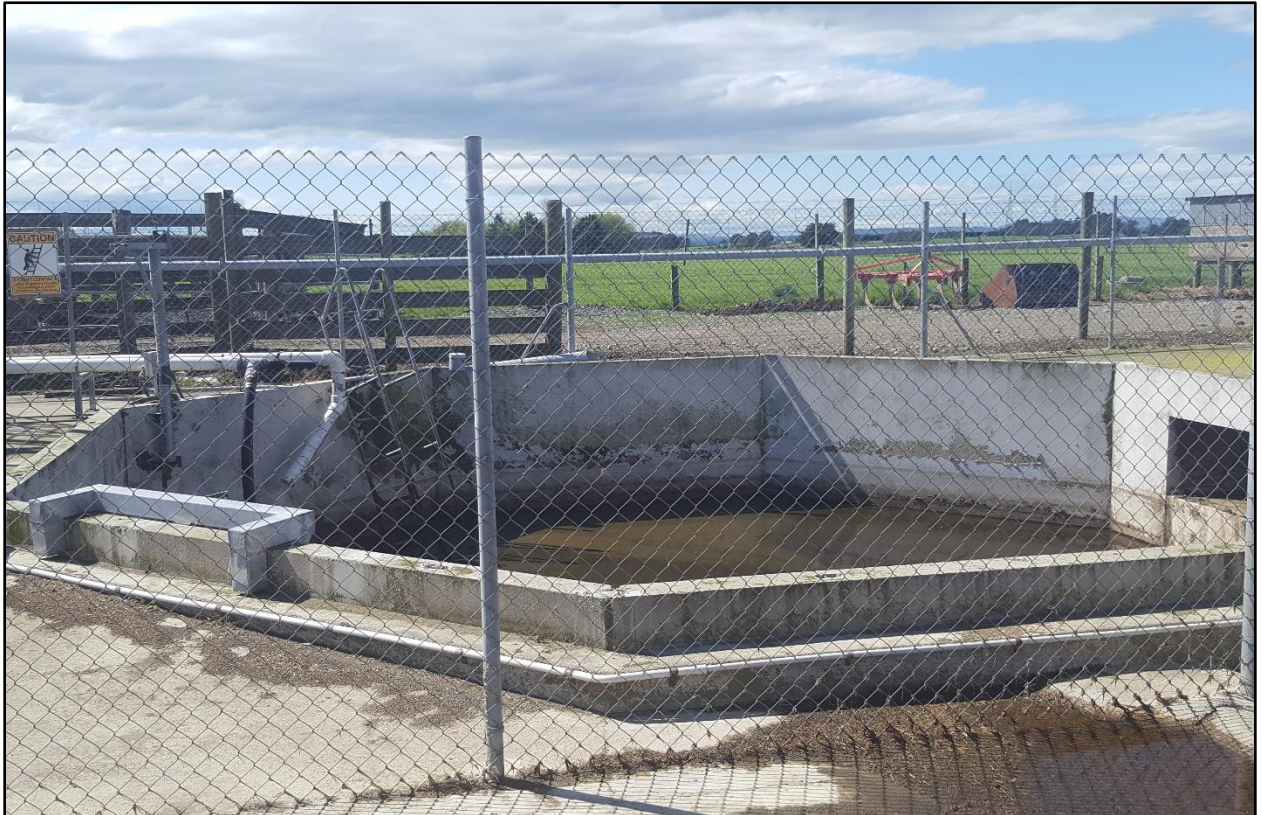
Figure 8: View of concrete sump (referred to a pump sump in Dairy Green Ltd reports attached)
