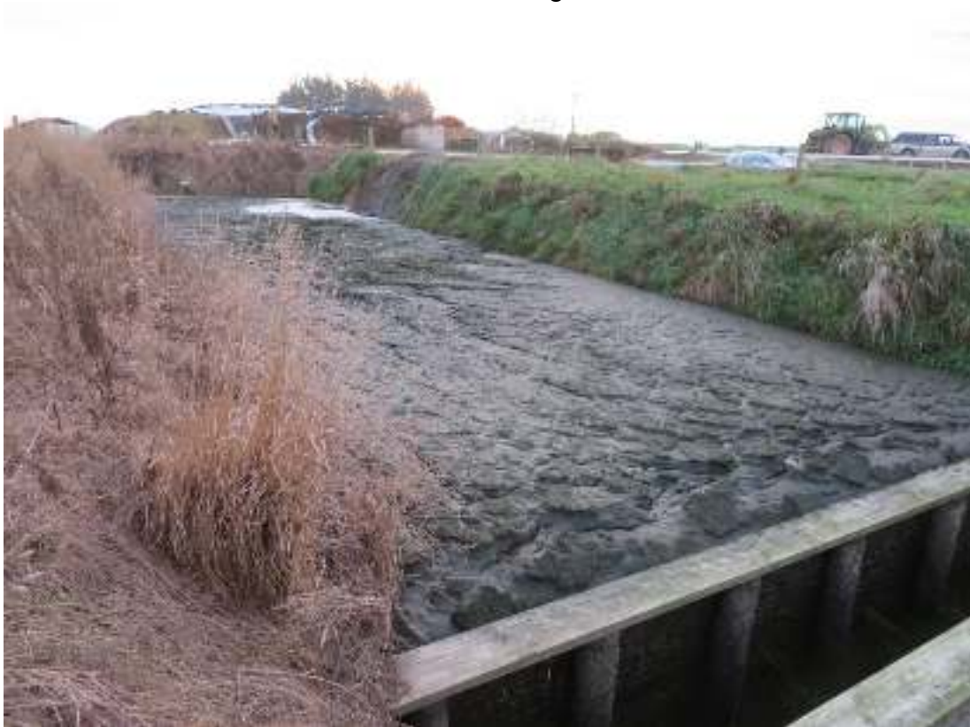
The western sludge bed.
