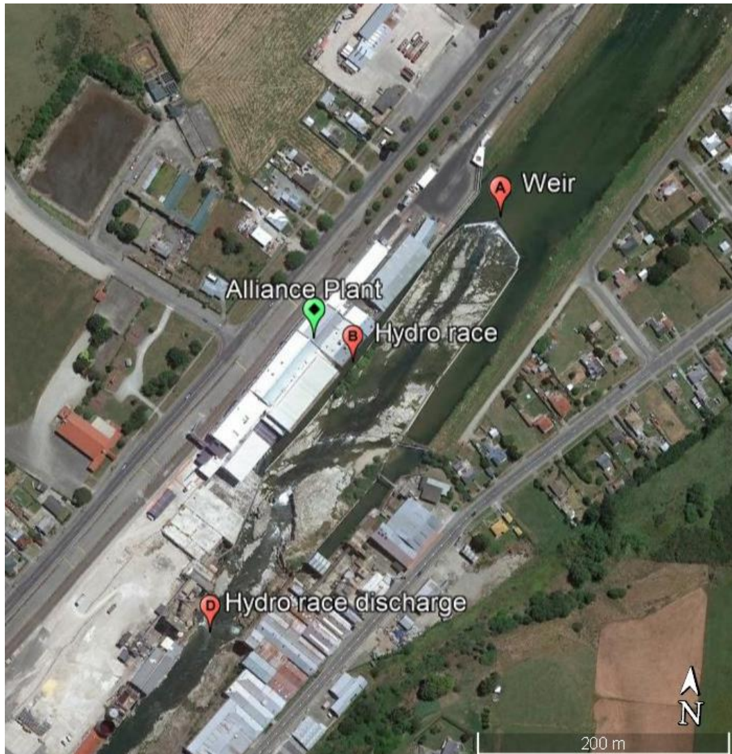
Figure 4: Weir, hydro race and discharge.
