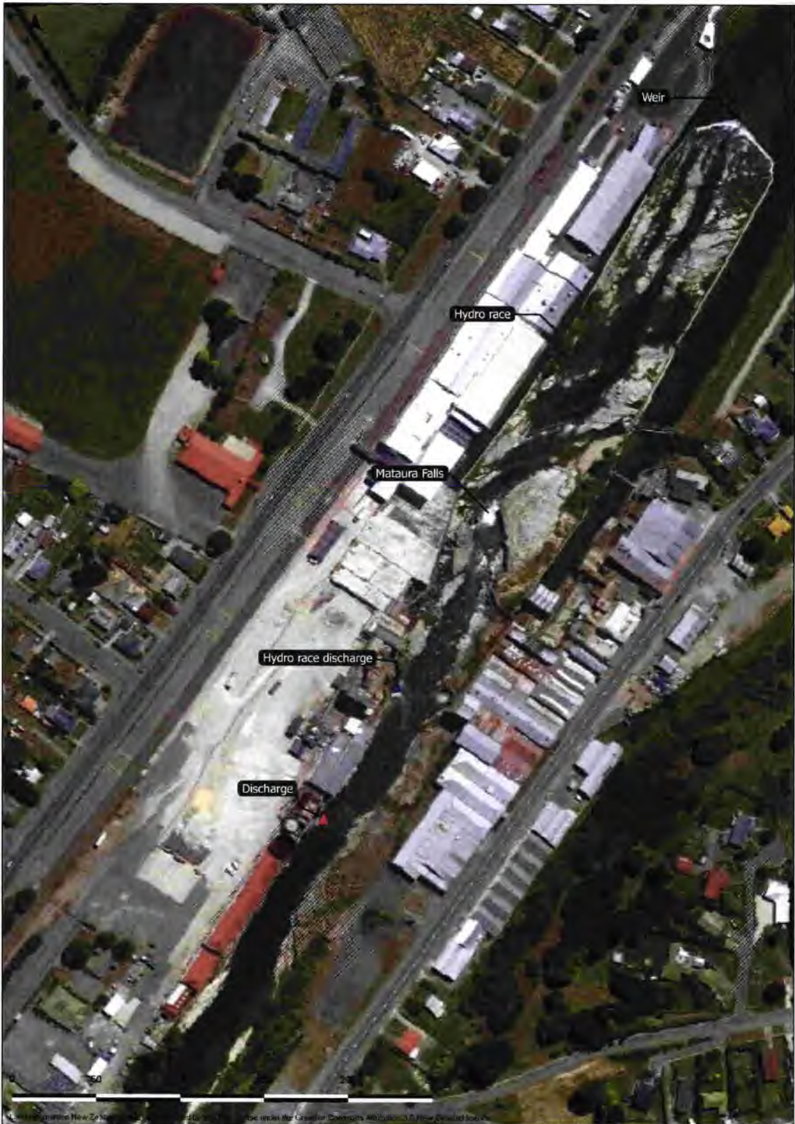
Figure 51: View of Matura River between the Matura Township Bridge and weir.
