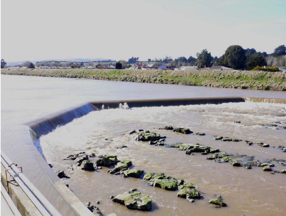
Fig. 2.2: The hydro-electric diversion weir and top end of the Alliance diversion raceway, note the shallow water over topping the hydro race along the side of race diversion wall.
