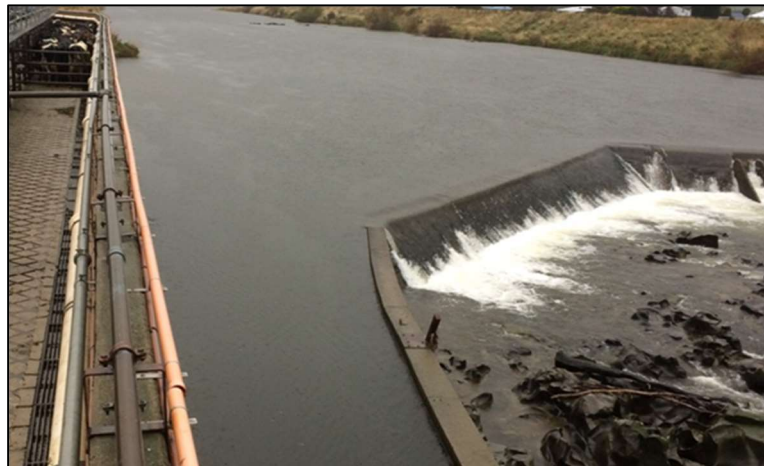
Figure 1 Flow over the broad crested weir apex
