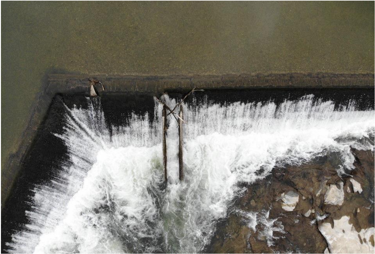
Figure 3. Drone photo view of top of the ladder.
