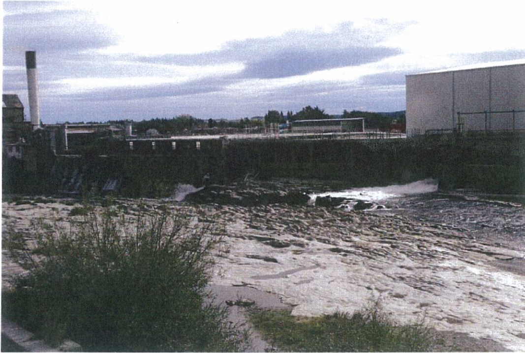
Figure 6. Alliance Matura showing flows from the headrace through sluice gates and overflows
