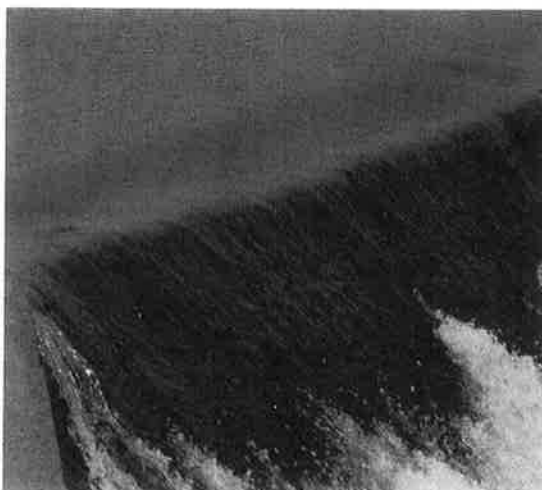
Figure 3A & 3B: Relationship between head upstream of a broad crested weir and depth of flow over the crest as occurs at low flow over the Mataura weir
