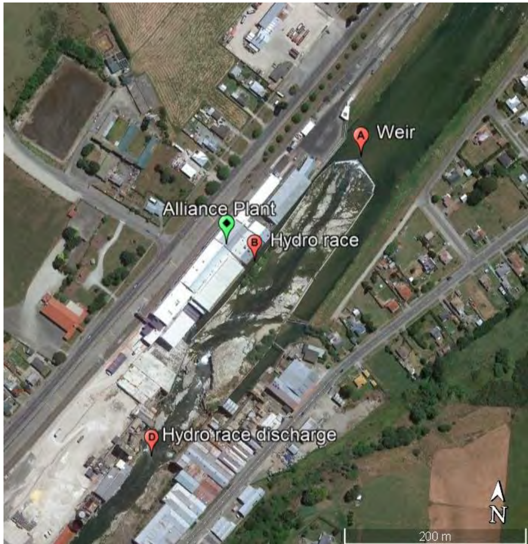
Figure 4: Weir, hydro race and discharge.
