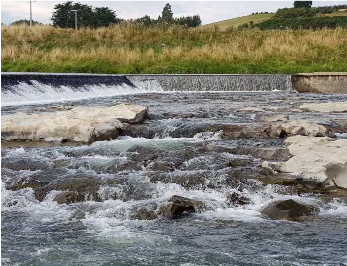
Figure 52: View of the weir and river environment immediately downstream.
