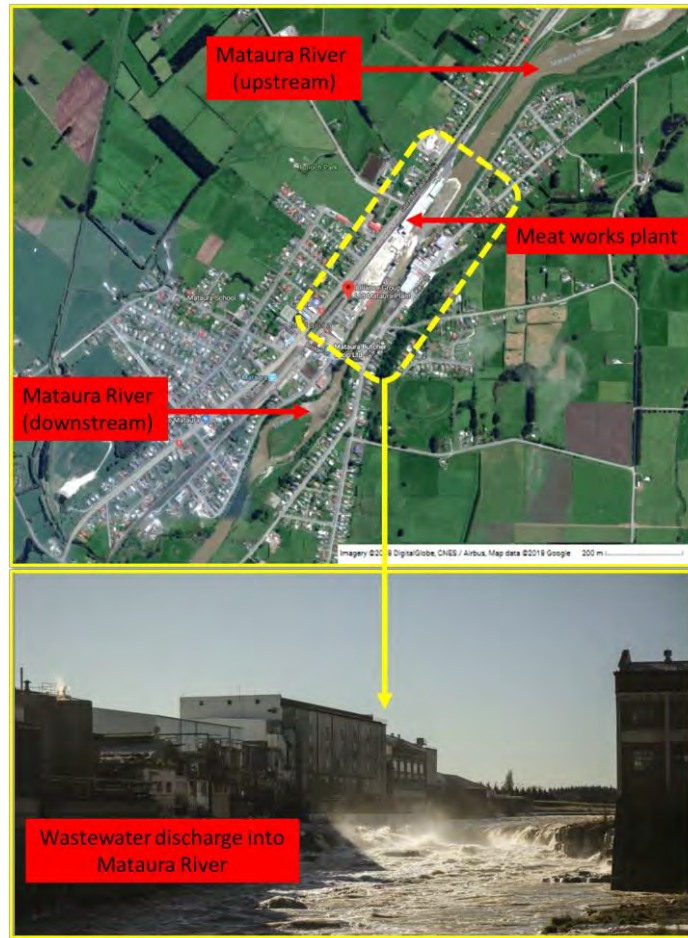
Figure 3 Physical location of meat processing factory and discharge of wastewater into the Mataura River
