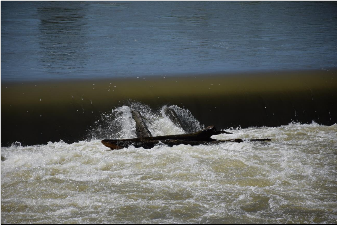
Plate 3: Weir fish ladder
