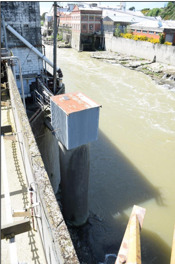
Plate 8: Wastewater discharge point
