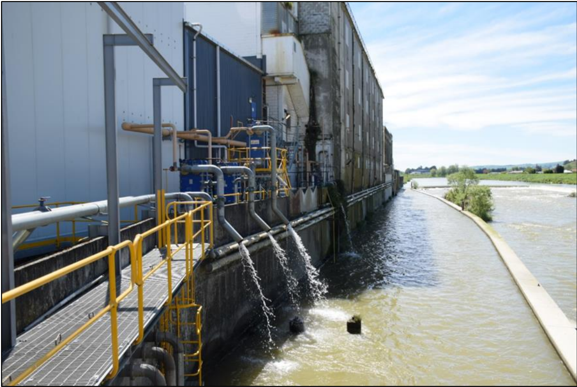
Plate 5: Cooling water discharge and hydro-race
