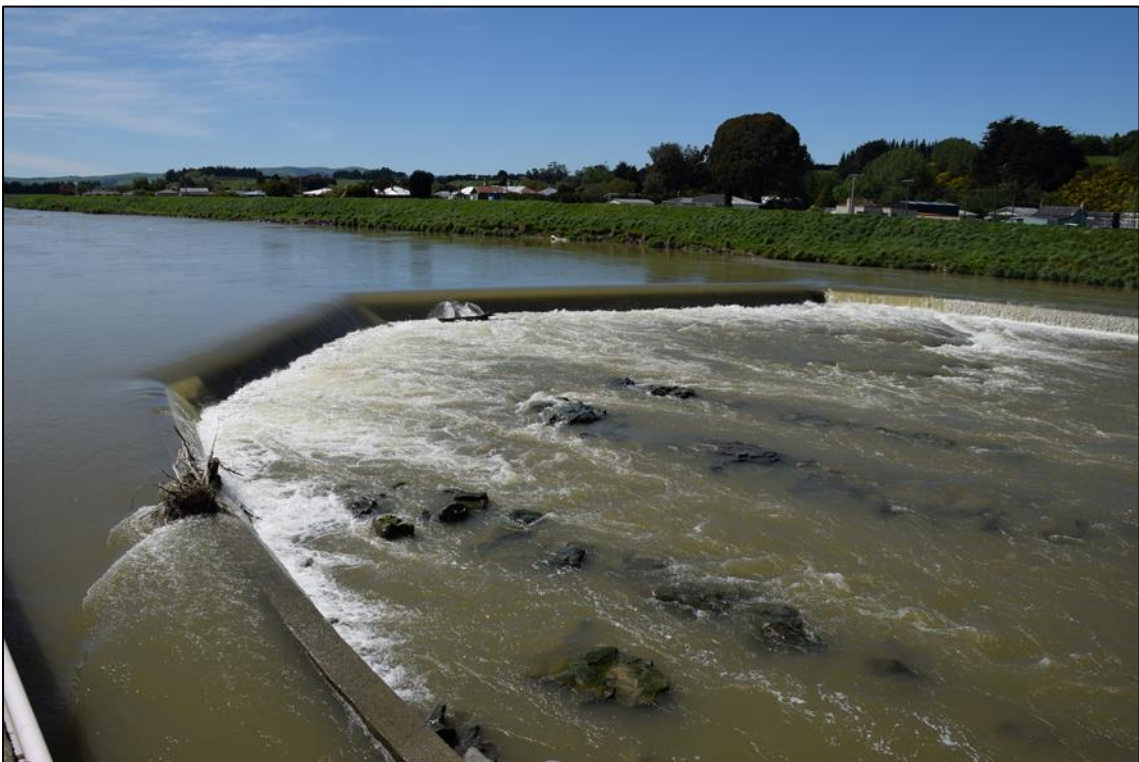
Plate 2: Weir from the Plant, showing the hydro-race in left foreground
