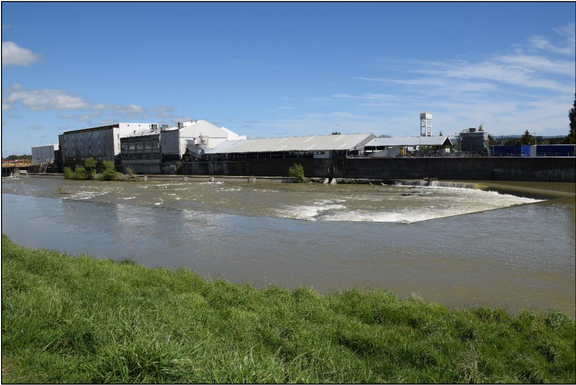
Plate 1: Plant and weir
