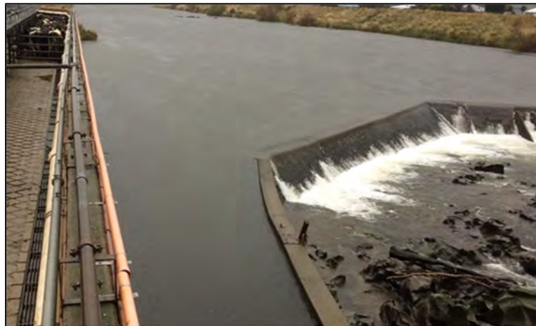
Figure 1 Flow over the broad crested weir apex
