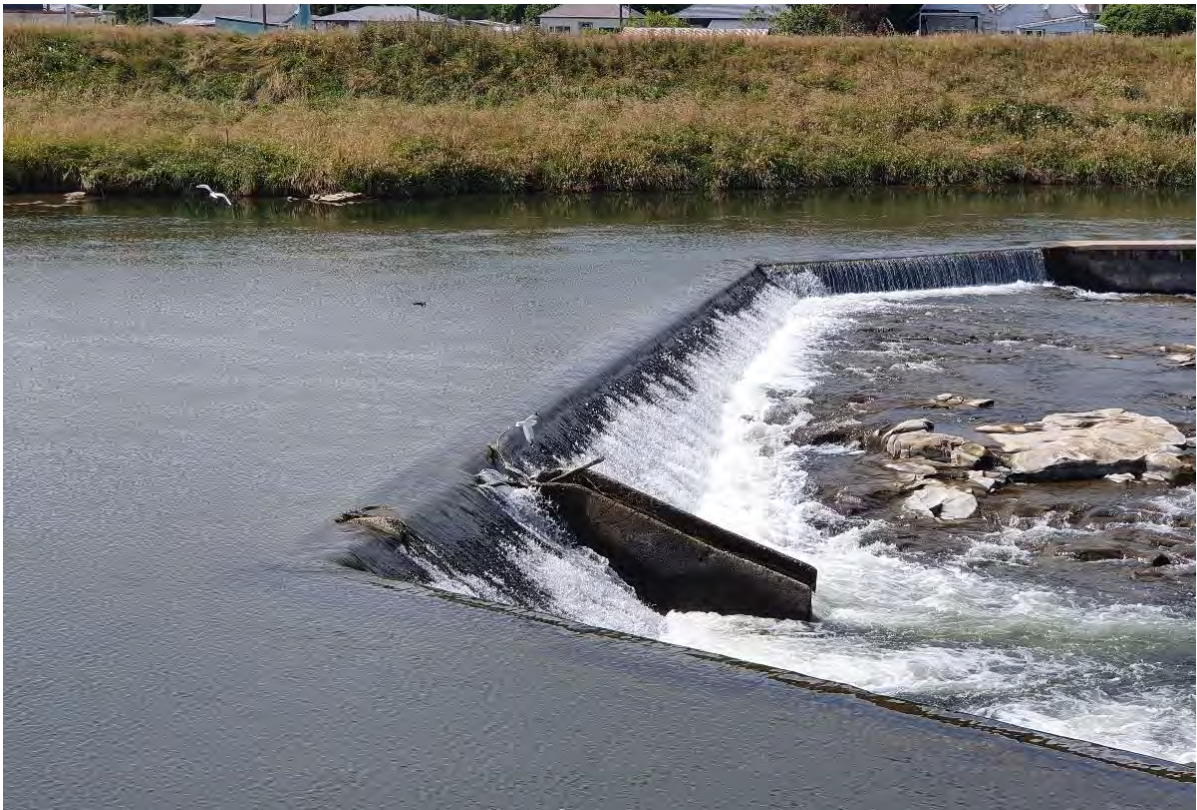
Figure 2. Fish ladder looking across to the true-left bank.
