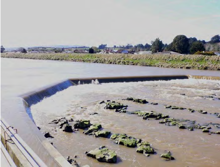
Fig. 2.2: The hydro-electric diversion weir and top end of the Alliance diversion raceway, note the shallow water over topping the hydro race along the side of race diversion wall.
