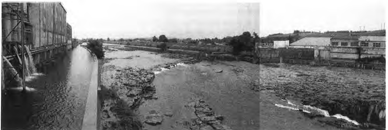
Figure 10: Panorama showing long weir crest from Alliance looking upstream
