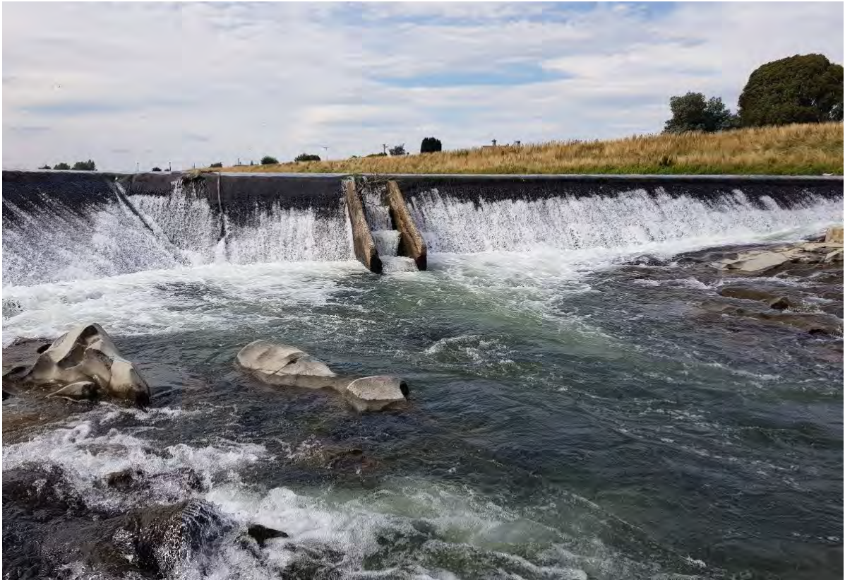
Figure 1. Pool and weir ladder at the Matura River Weir.
