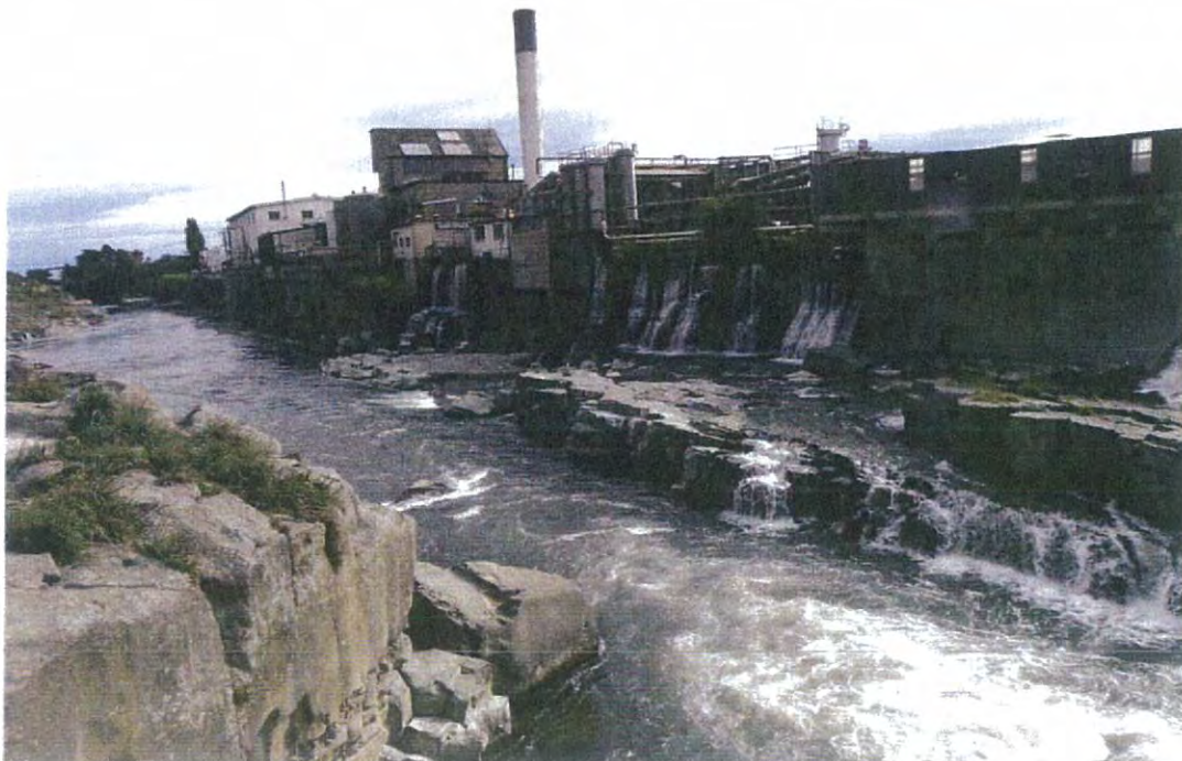
Figure 7. Alliance Matura downstream of the falls showing flows across the rock shelves as a result of the hydro race discharges
