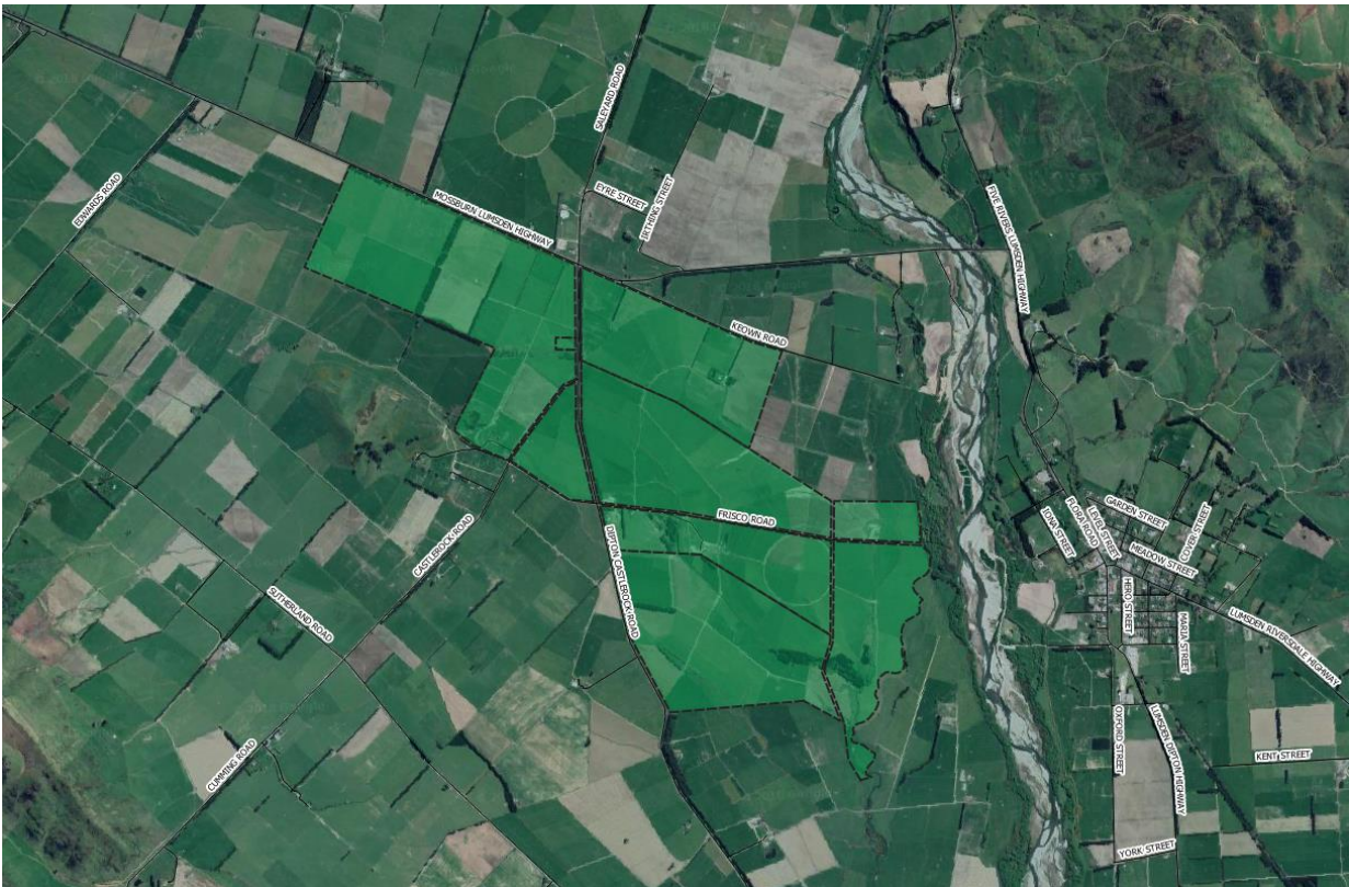
Figure 1 - The site is located on the opposite (western) side of the Ōreti River from the town of Lumsden.
