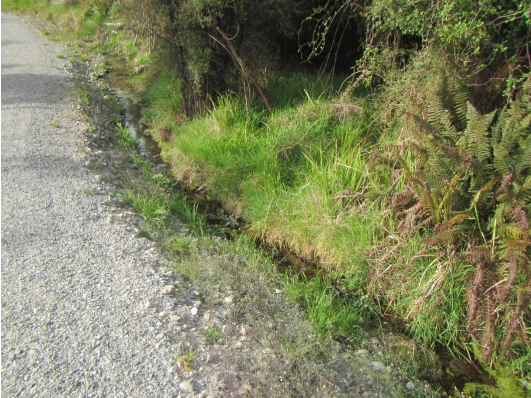
Plate 5: The excavated ditch on the upstream side of the cycle trail that is resulting in adverse hydrological effects on the upstream wetland. 4 November 2019.
