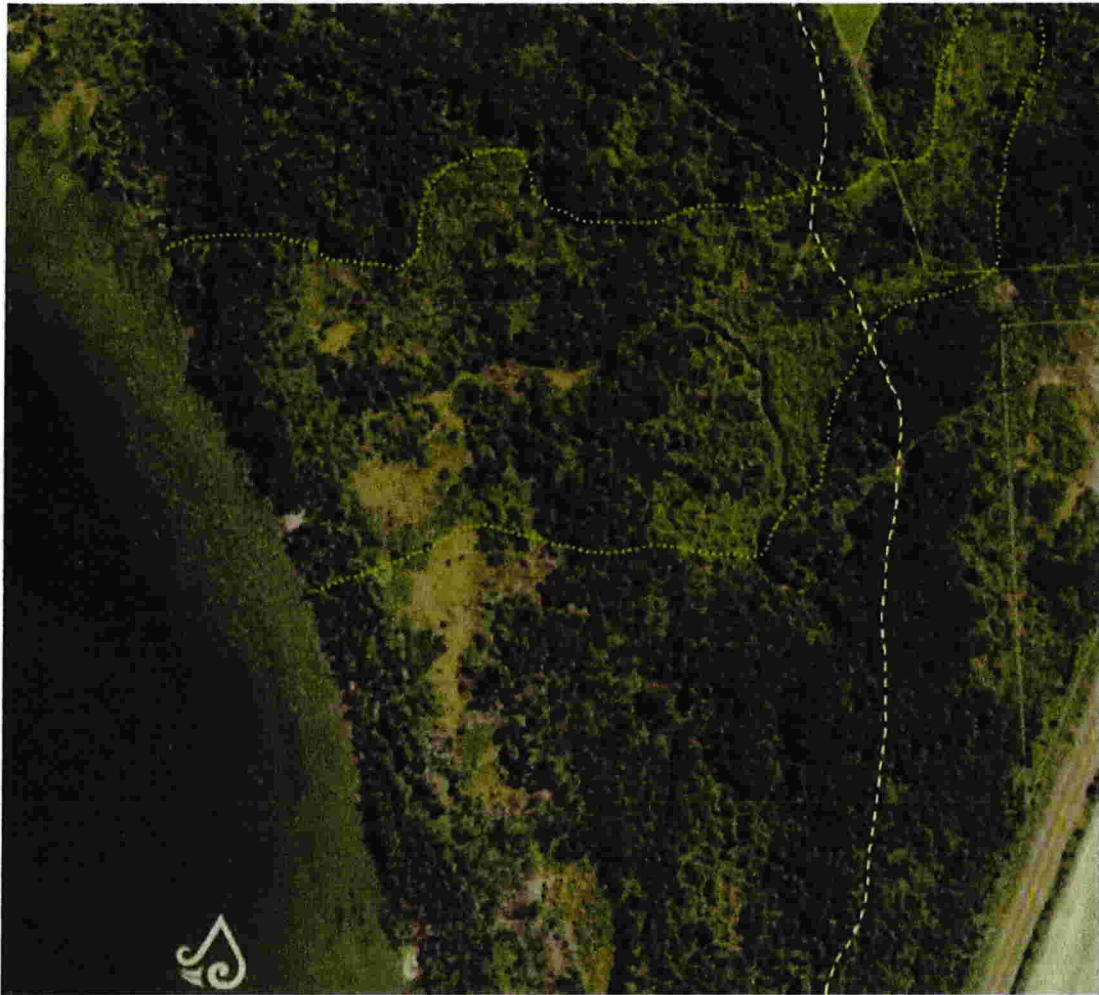
Figure 8-1: Aerial extracted from Southland District maps depicting trail alignment in context to the wetland.
