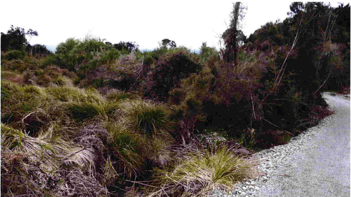
Figure 5-2: Extensive sedgeland of purei downstream of the southern culvert.
