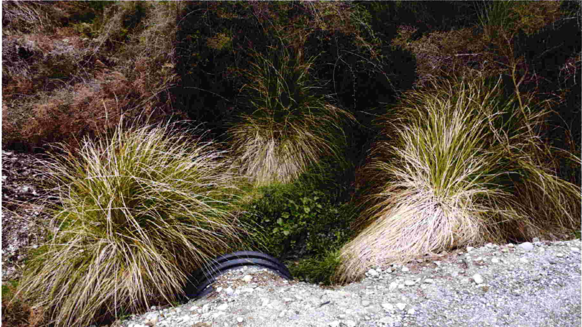
Figure 5-1: Purei bordering the inlet to the northern culvert.
