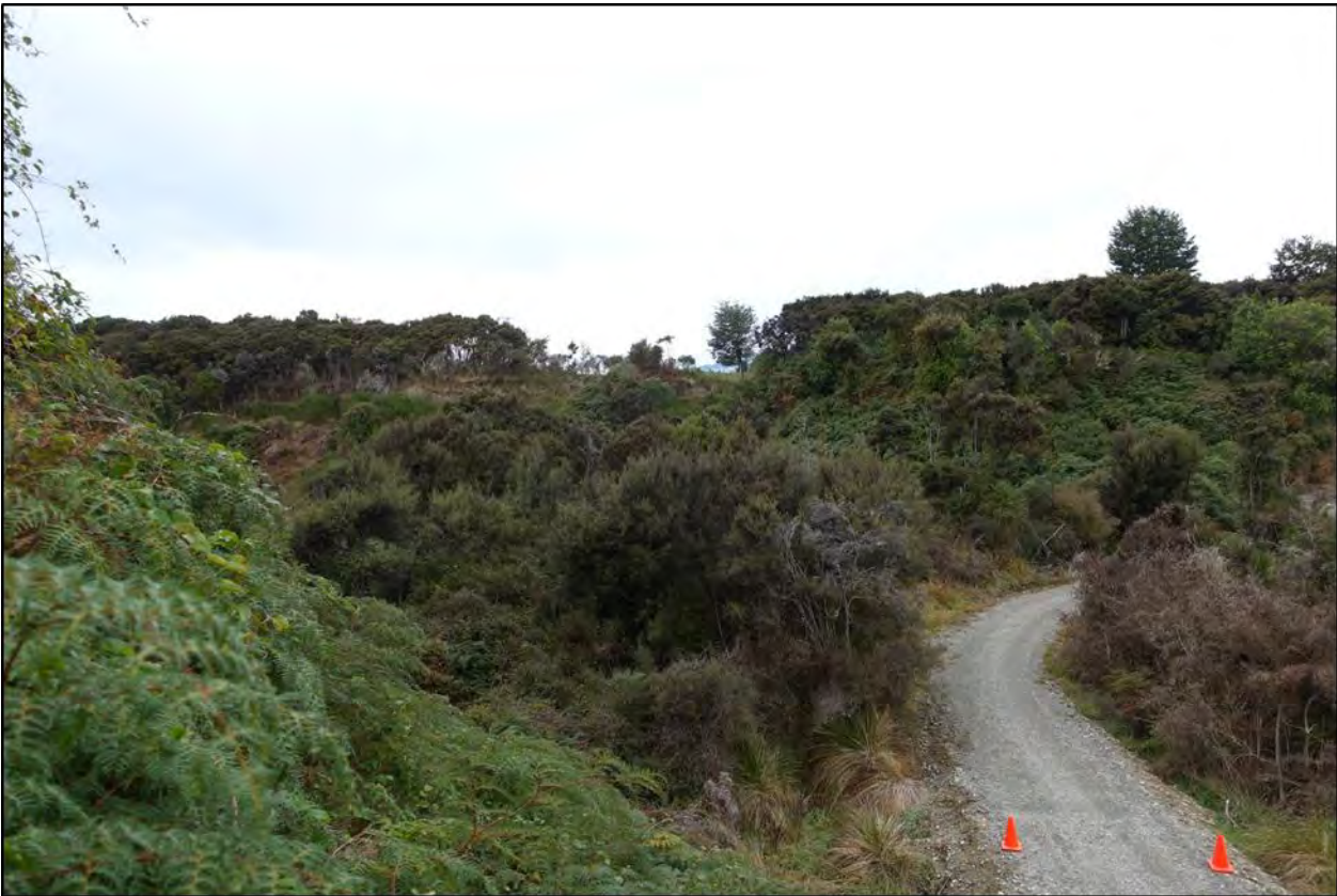
Overview of the area upstream (east) of cycle trail. The road cones mark the position of the northern culvert.
