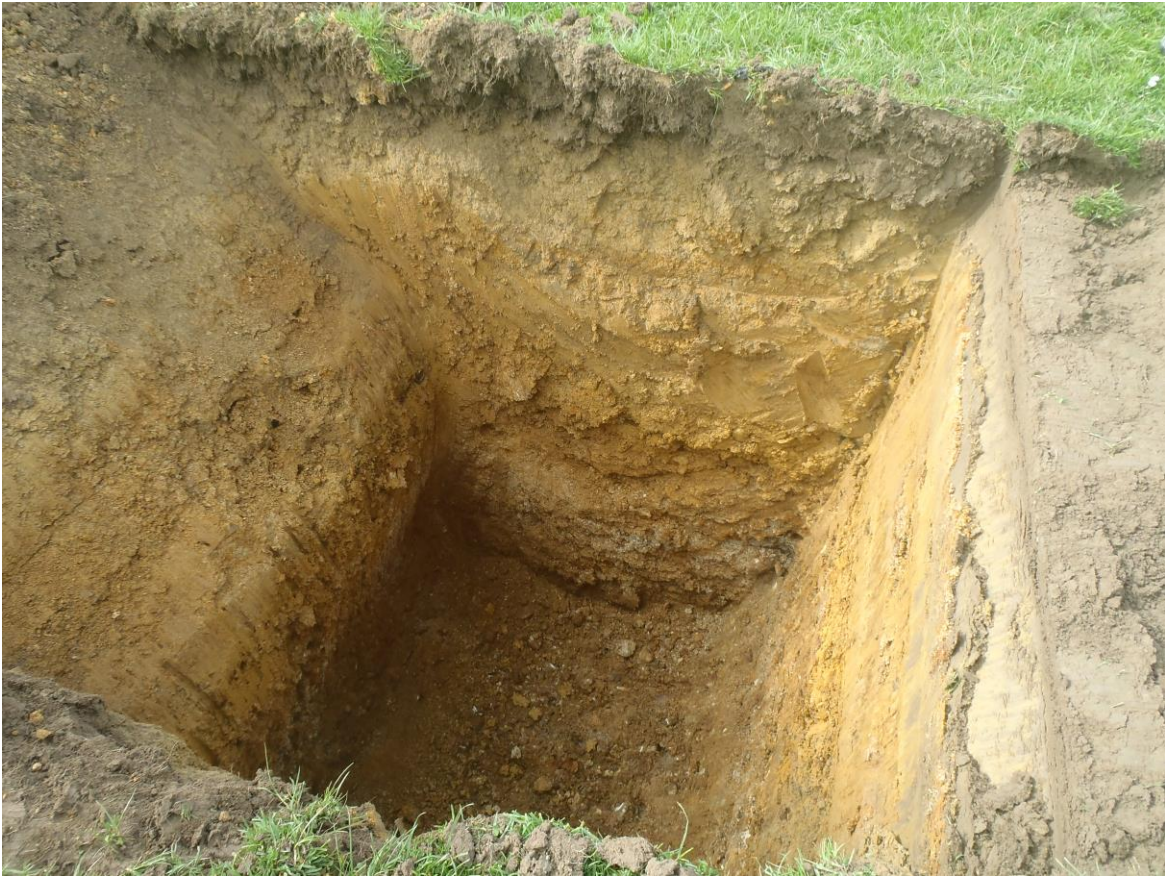
Test Pit Cut
