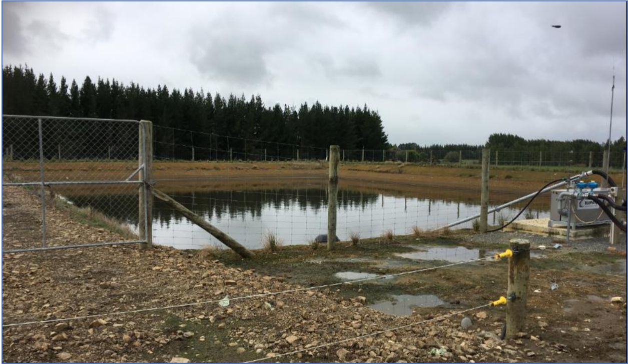
Figure 4: Effluent Pond, which is fully fenced
