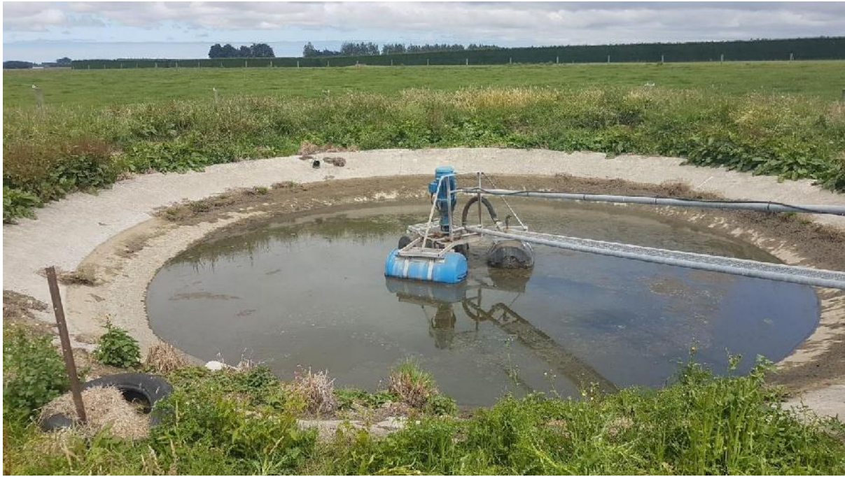
Figure 21: Concrete saucer on SD2
