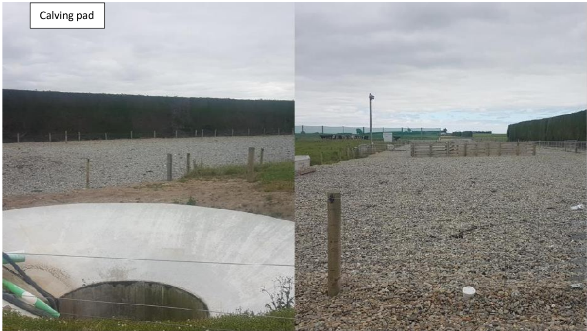
Figure 8: Calving pad with gravel base and connected concrete saucer at SD1
