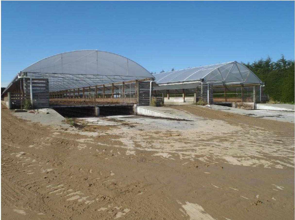
Looking east toward the twin Herd Homes and the under floor storage bunker.
