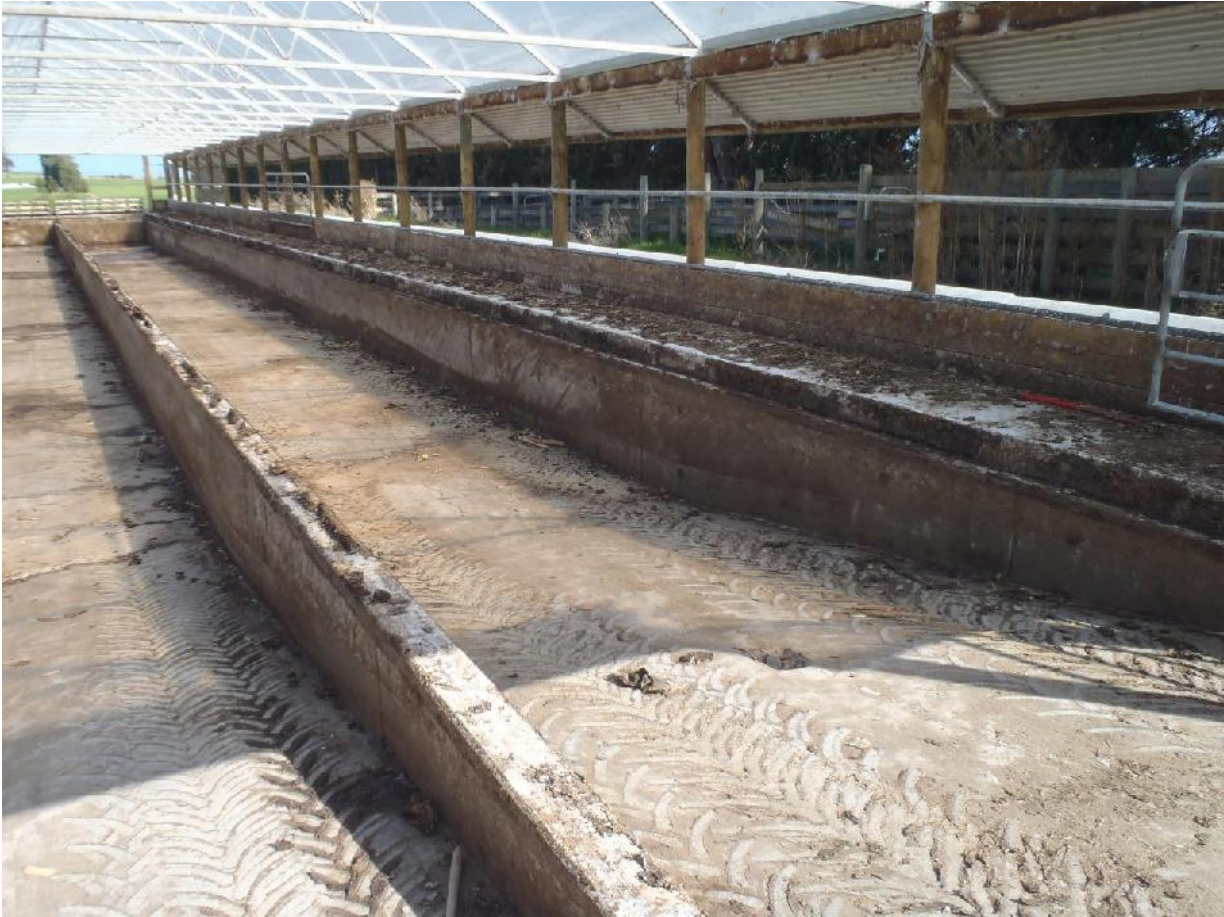
Looking south at the open west bunker.
