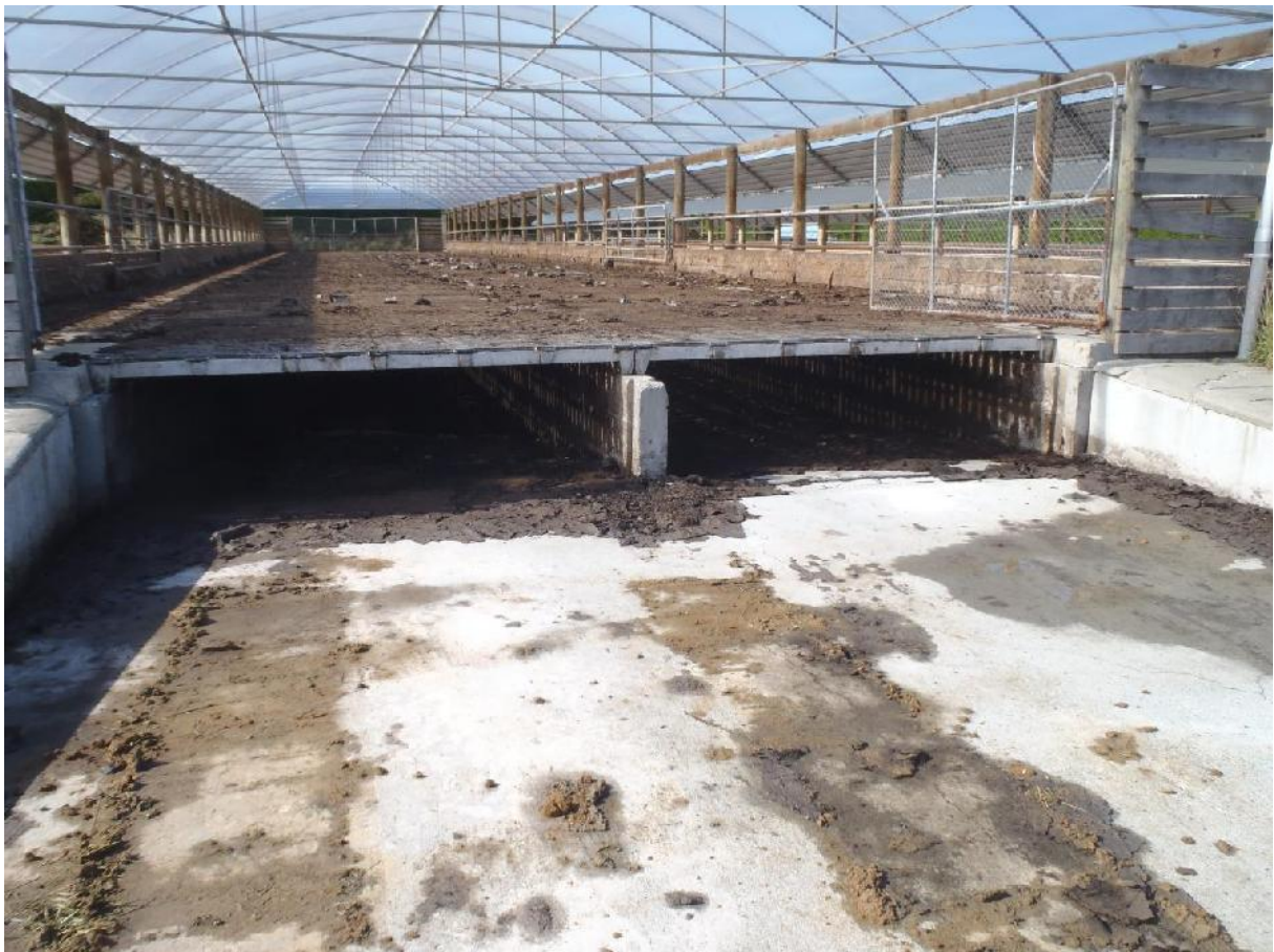
Looking east into the under floor storage bunker.
