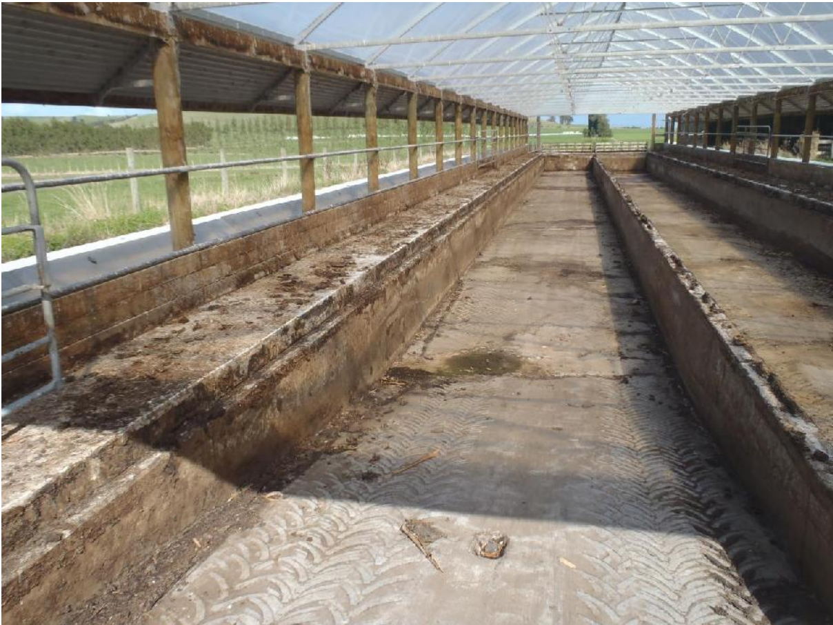
Looking south at the open east bunker.
