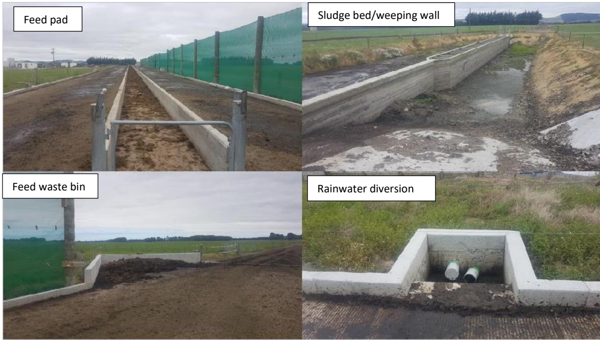
Figure 7: Images of feed pad and connected effluent structures at SD1
