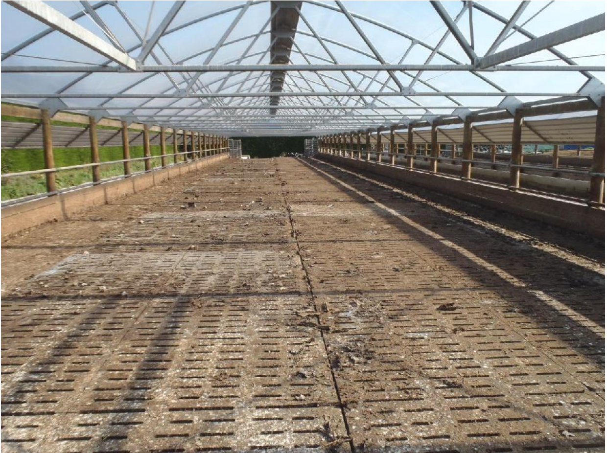
Looking west along the slotted floor above the storage bunker.
