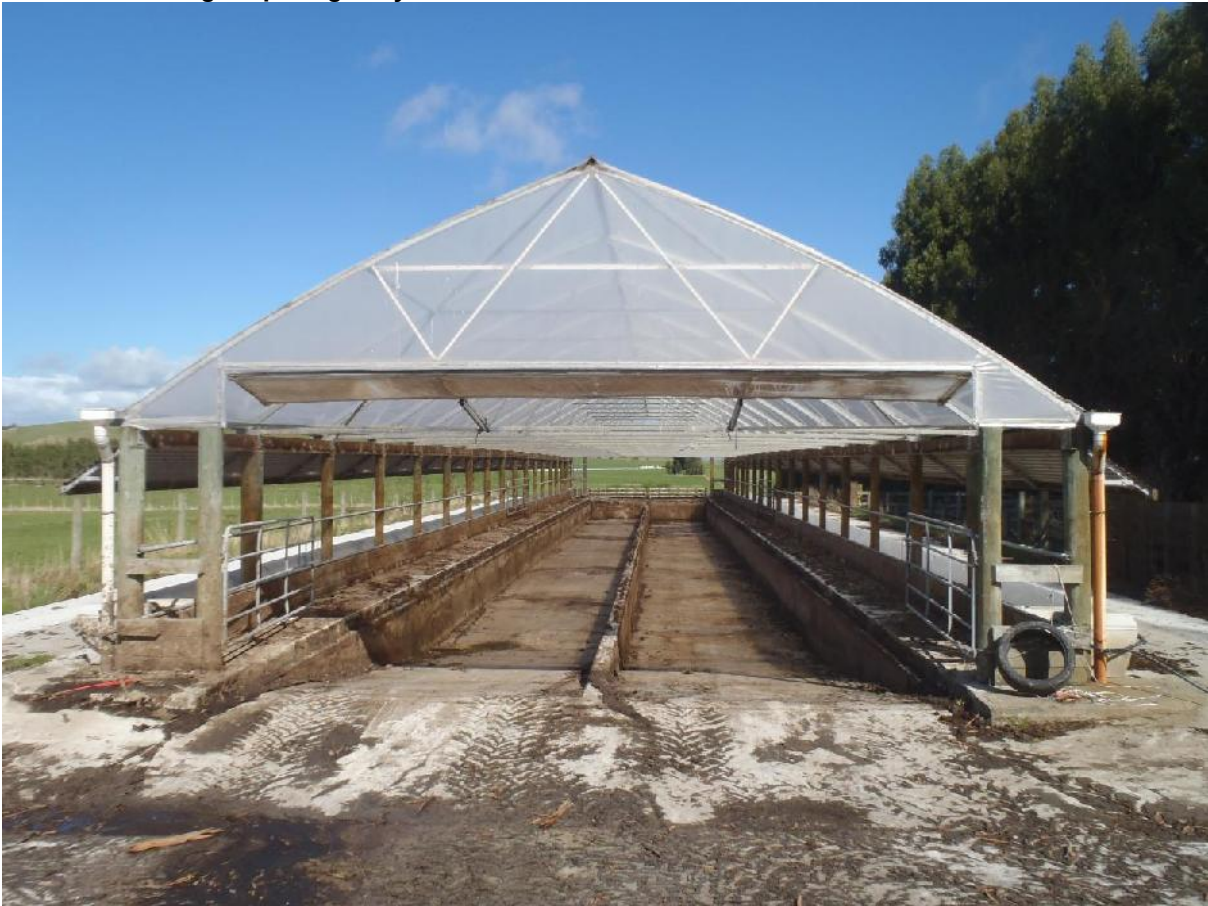
Looking south at the open effluent storage bunker.
