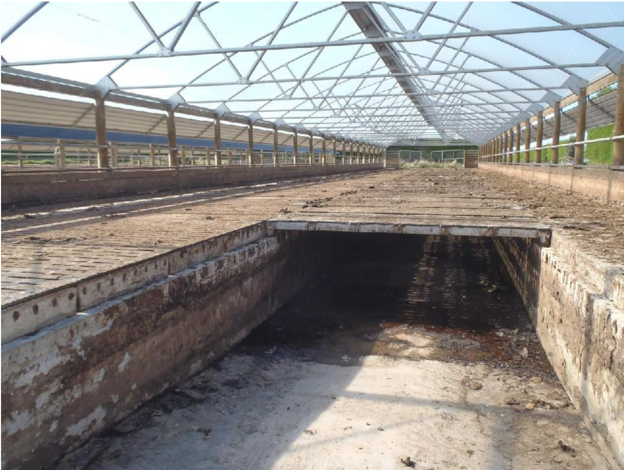
Looking east at the storage bunker.
