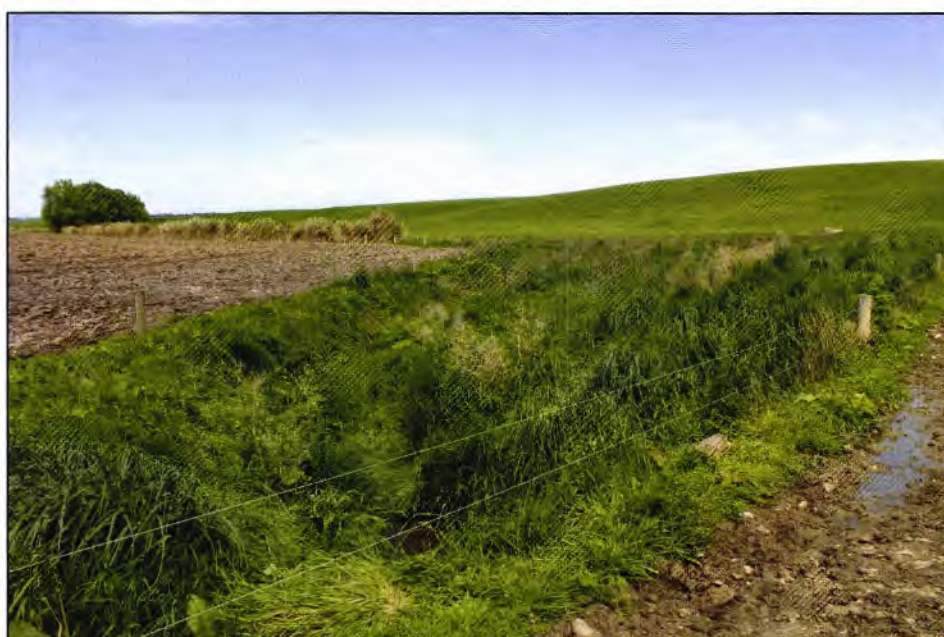
Figure 7.3 Photo of fenced-off, well vegetated culvert CSA.
