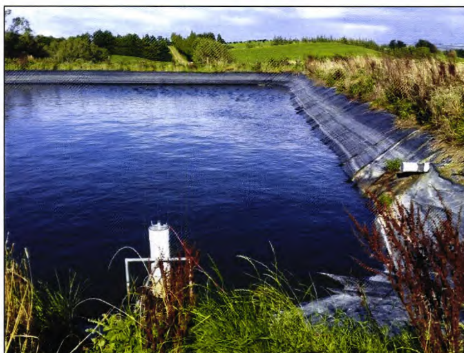
Figure 6.5 Effluent storage pond
