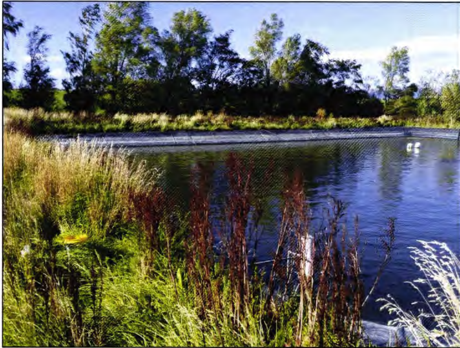
Figure 6.6 Effluent storage pond
