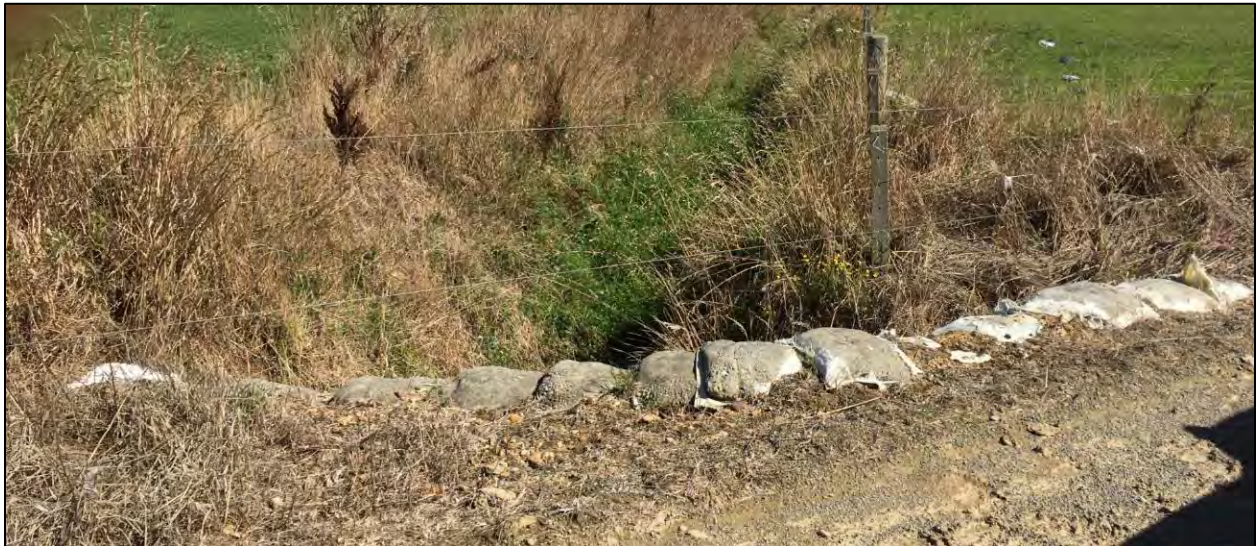
Figure 20: Laneway crossing with sandbags to prevent direct runoff into creek
