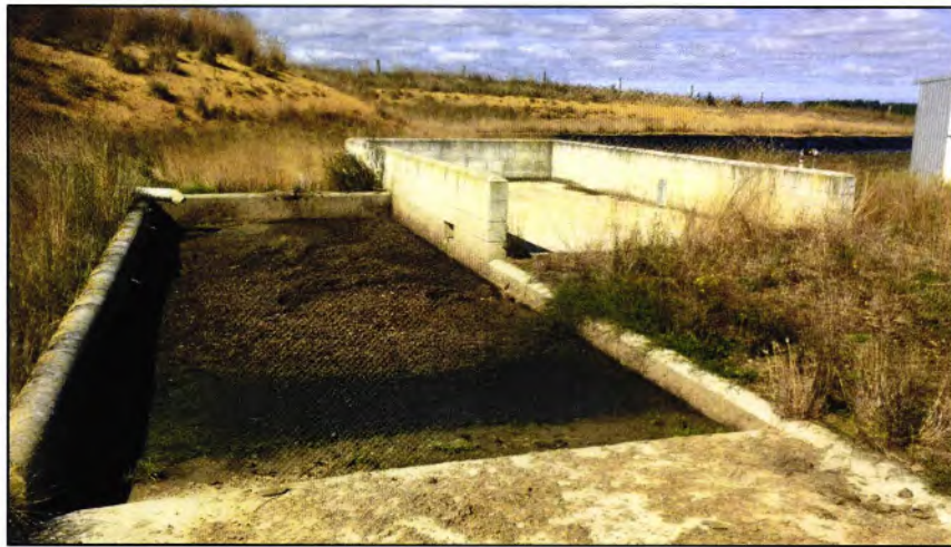
Figure 3: Large stone trap adjacent the effluent pond
