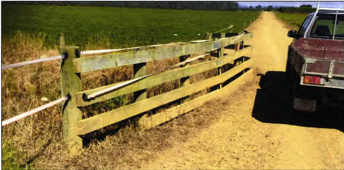
Figure 9: Laneway crossing with kickboard to prevent direct runoff into creek
