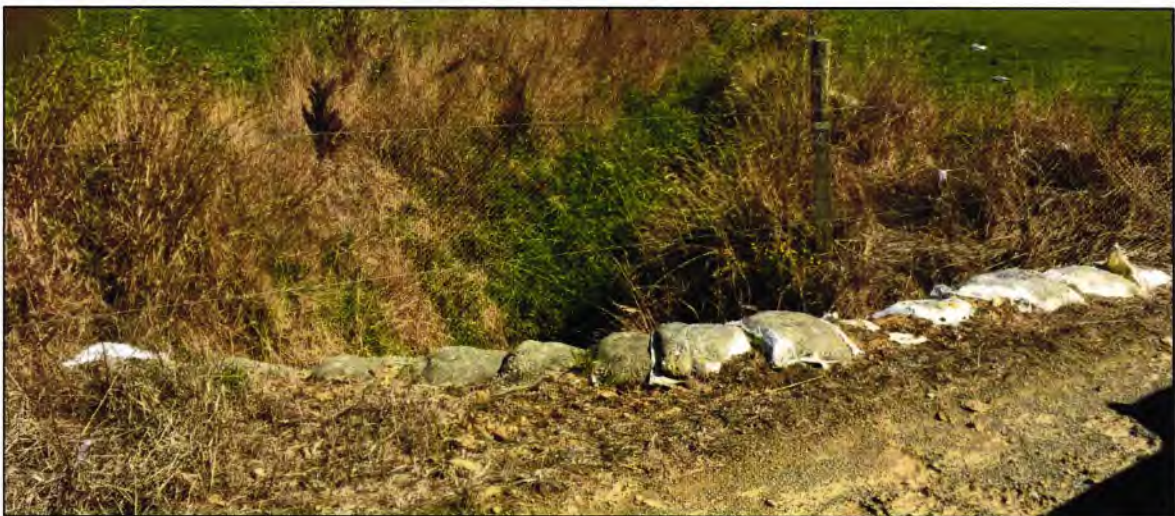
Figure 11: Laneway crossing with sandbags to prevent direct runoff into creek
