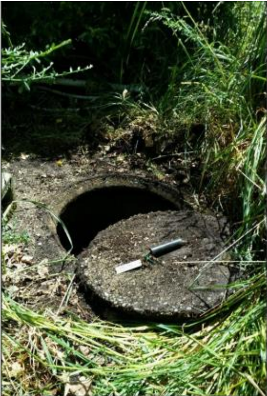
Bore E45/0622 before and after remediation by Southdrill
