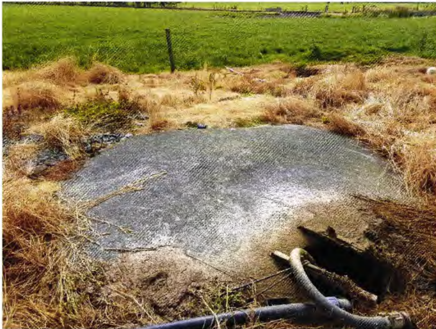
Figure 17: Photograph of existing pump sump
