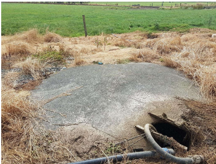
Figure 17: Photograph of existing pump sump
