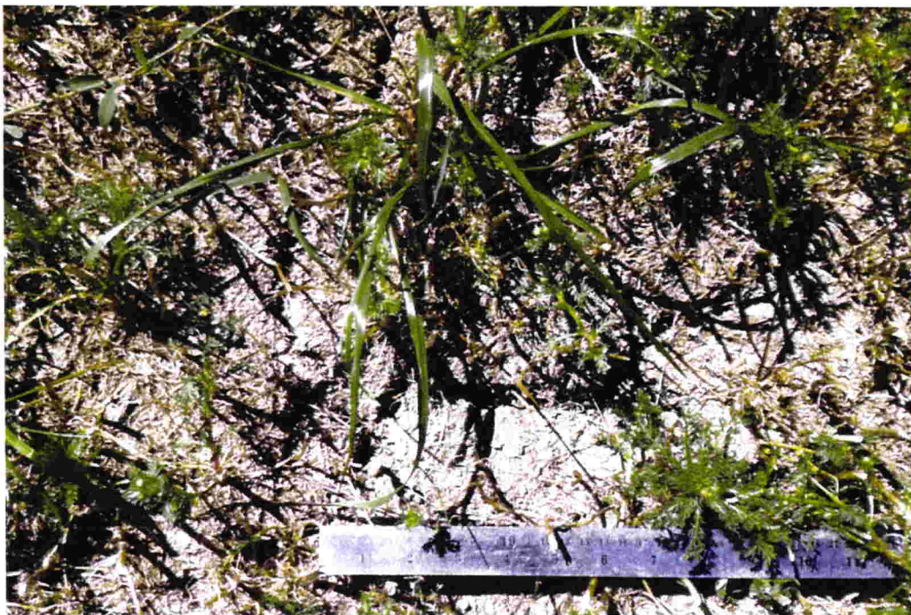
Figure 1. Cracked soil at Site 1.
