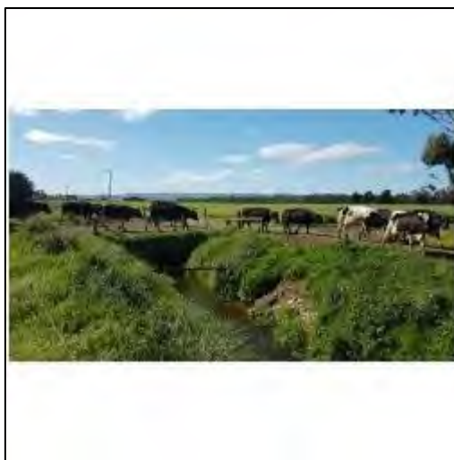
Figure 6.10 Cows crossing waterway over culvert to walk to the dairy shed on the east lane. Please note the wide buffers with long grass flanking the stream on both sides.
