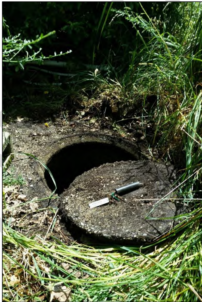
Figure 5.29 WOL bore (E45/0622) used for groundwater quality monitoring.
