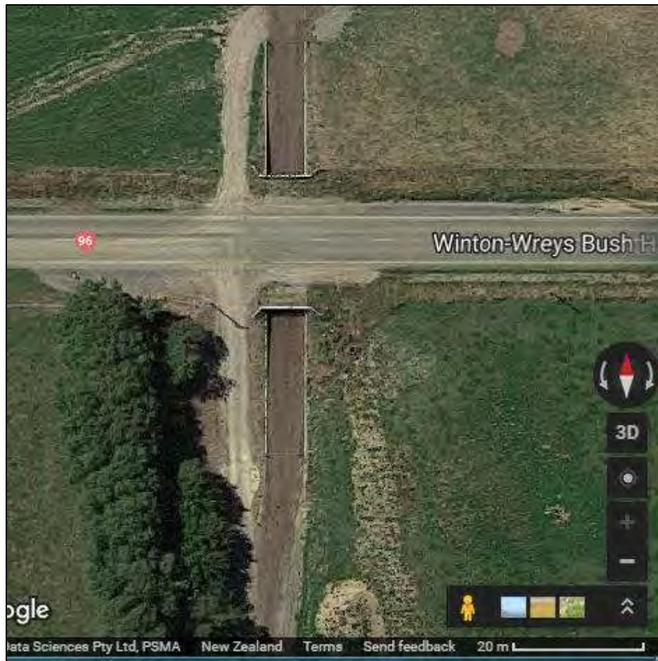
Figure 6.3 Aerial photograph of underpass.
