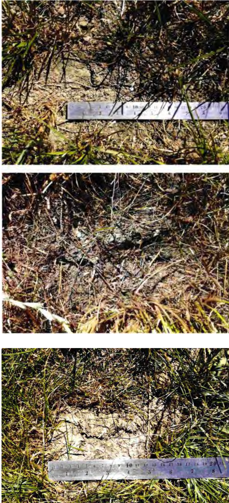
Figure 1 Images of soil cracks Killick, M (2018)
