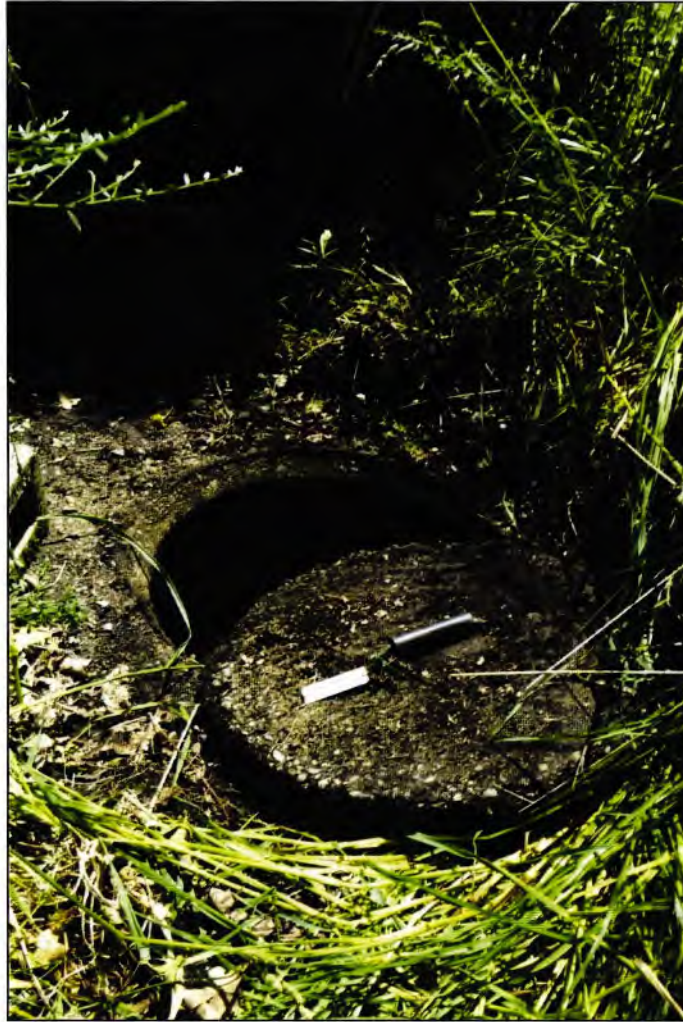
Figure 5.30 WW1 bore (E45/0622) used for groundwater quality monitoring.
