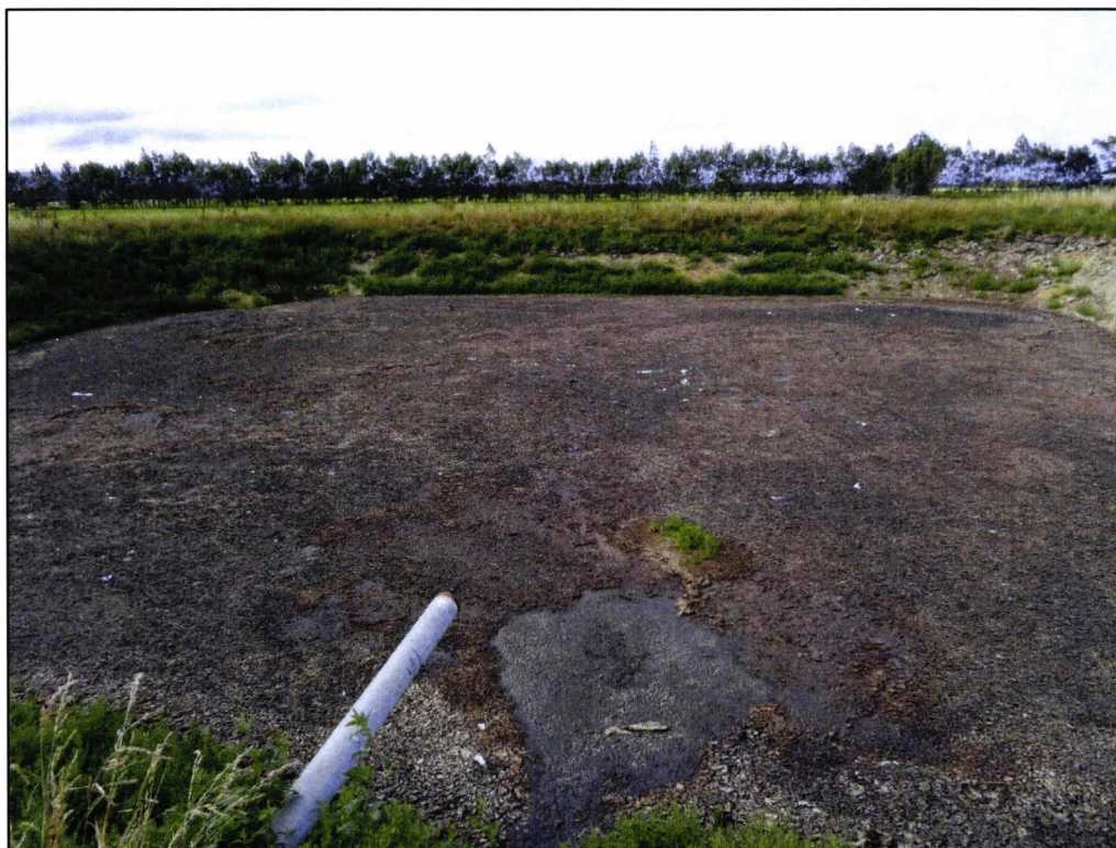
Figure 3. Photo of WW2's effluent storage pond.
