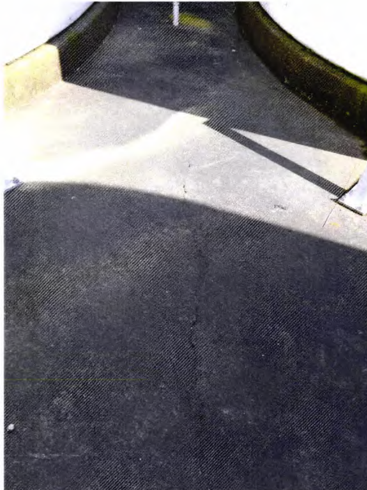
Cracking to Bund Floor
