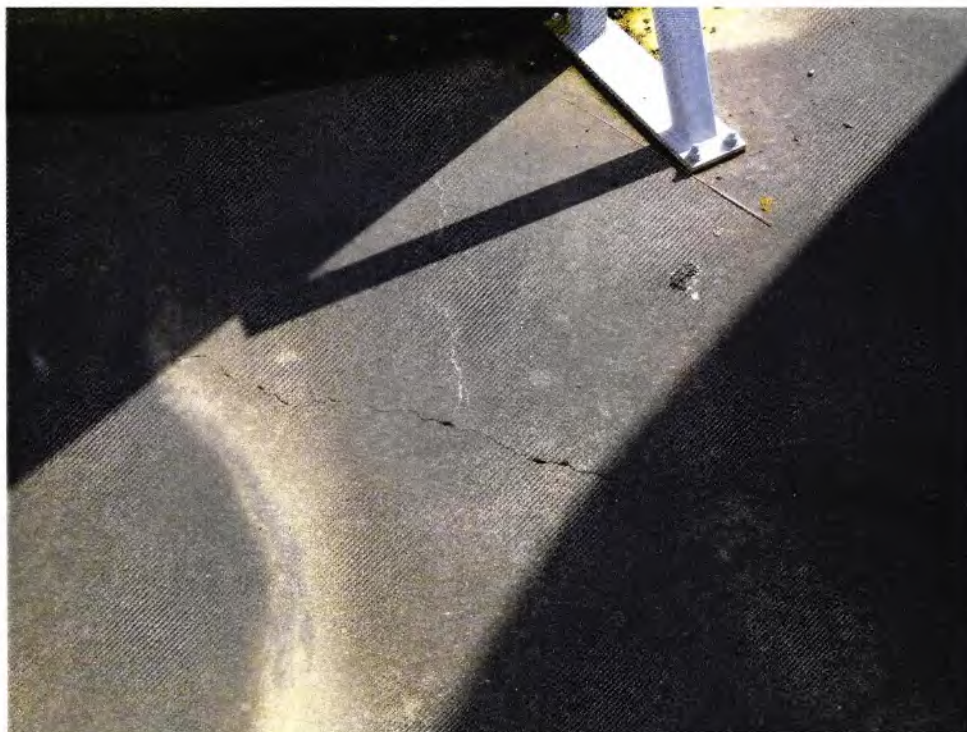
Cracking to Bund Floor
