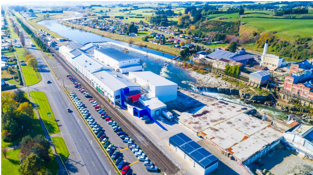
Figure 1: The Alliance Mataura Meat Processing Plant (foreground).
