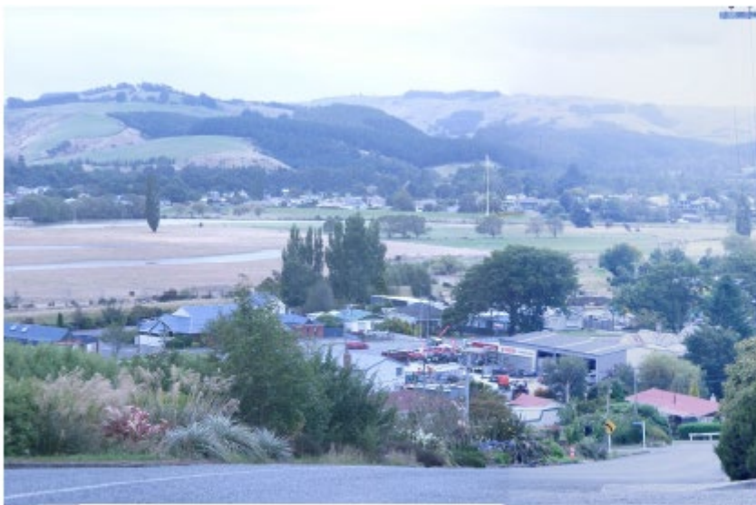
Figure 15: Viewpoint 4 - The viewpoint from the corner of Norton Street and Garnet Street post development. The bridge links the urban areas, however the structure is within context
