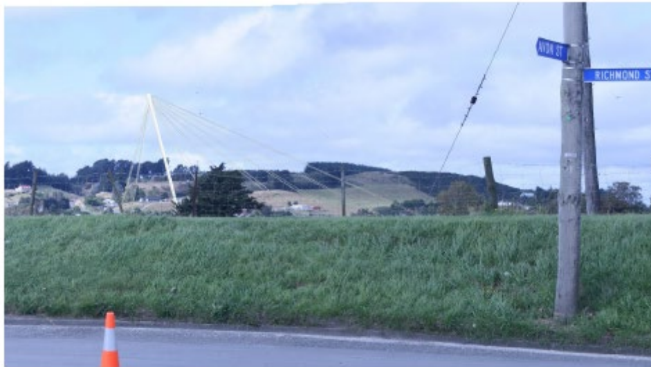
Figure 9: Viewpoint 1 – Post development. Showing the proposed bridge structure visible behind the stop banks.
