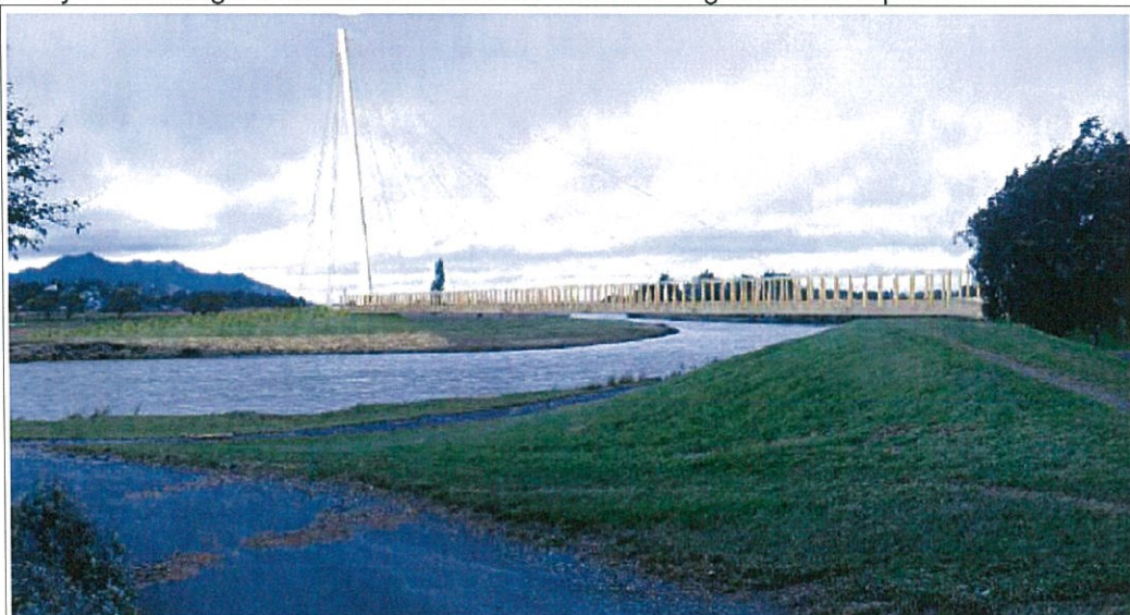
Figure 13: Viewpoint 3 - The viewpoint from the corner of River Terrace and Huron Street post development.
